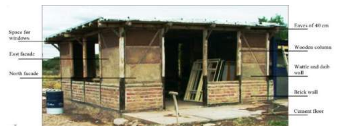
Fig. 11. Workshop construction stage.
