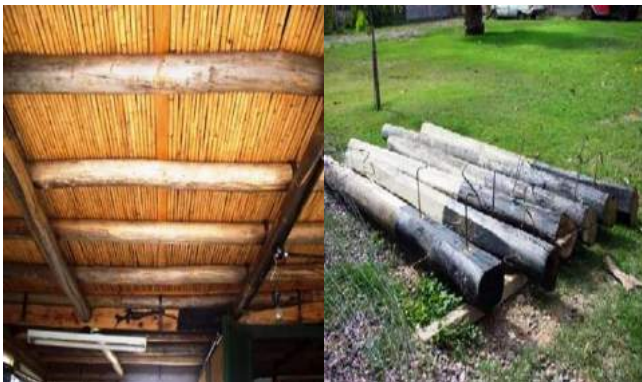
Fig. 8. a-Cane roof and b- Eucalyptus wood columns.
