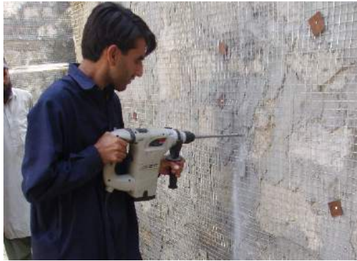
Drilling holes for the bolts
