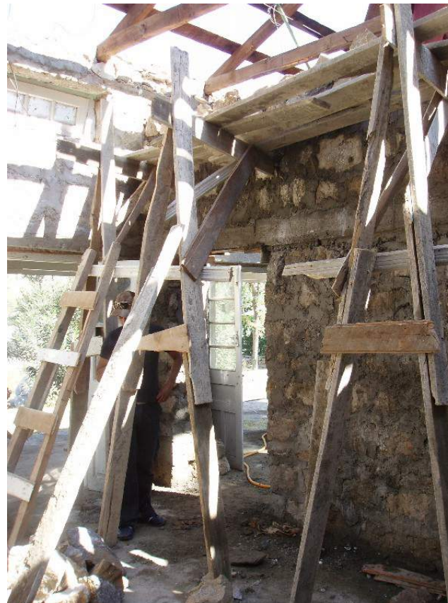
New wall with lintel
