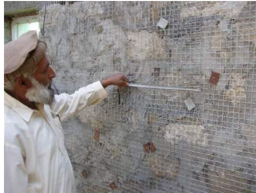
Wire meshes have to overlap 1'
