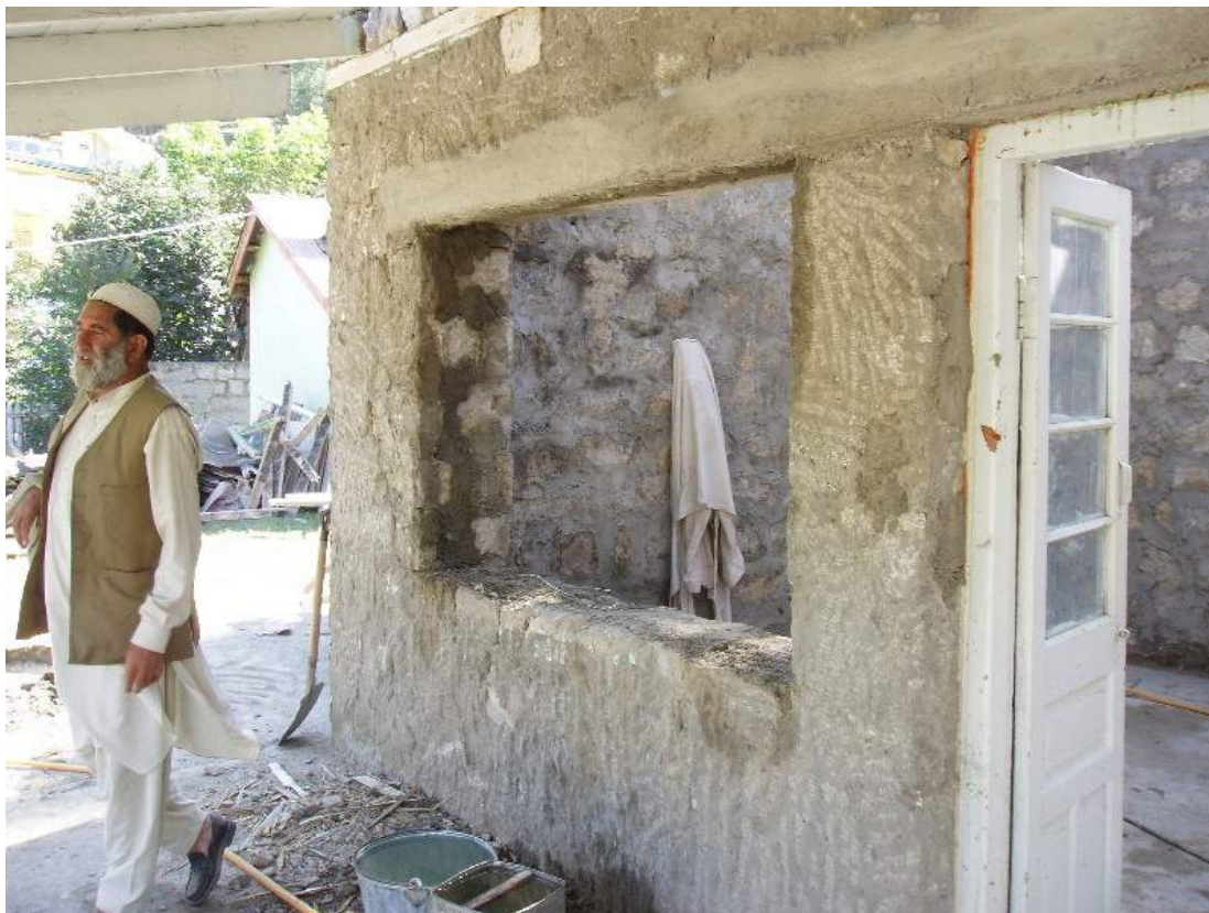
Replaced lintels above door and window
