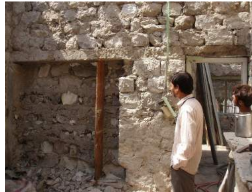
Cupboard niche in wall
