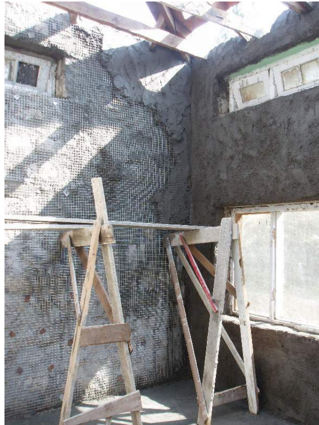
Cover of mesh with plaster
