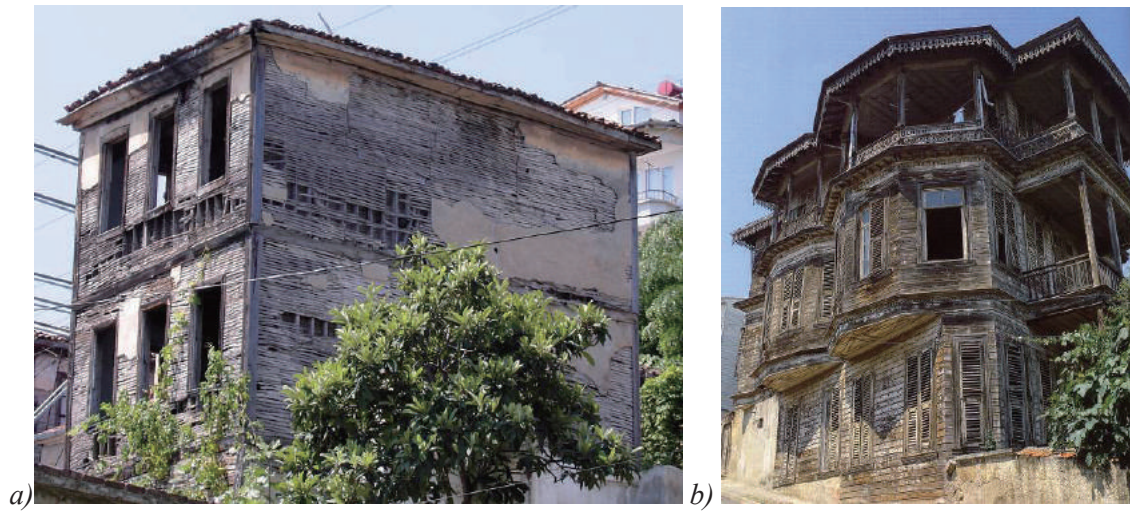
Fig. 4: Timber covered frames
