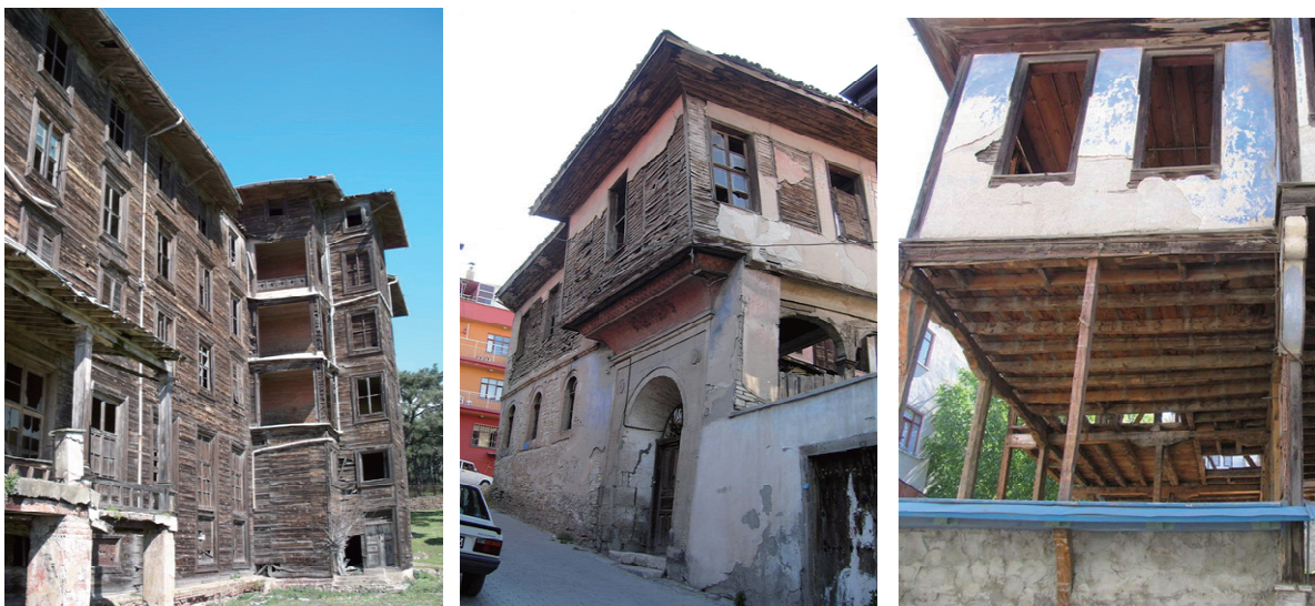
Fig. 2: Timber houses rise on foundation wall, on masonry wall and on columns
