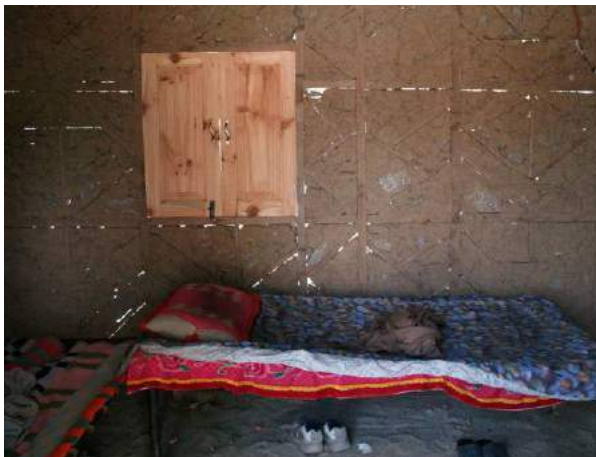
Figure 13a: Infills should mainly be of stones with a limited amount of mud.
