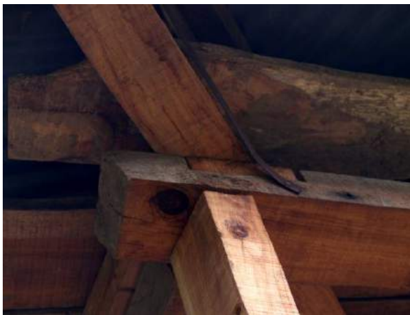
Figure 6f: insufficiently strong corner connection (hold only through vertical nails)
