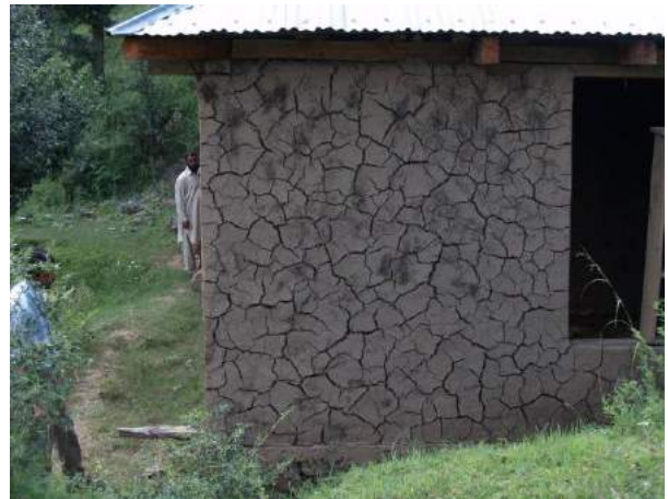
Figure 14b: excessive thickness of a single plaster layer results in cracking.
