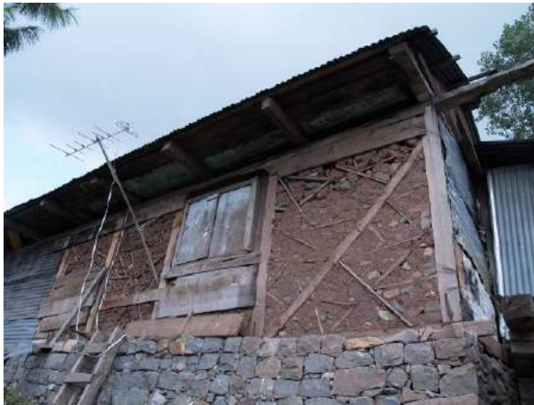
Figure 4c: Irregular fill-in with long corner braces, creating an imbalance.
