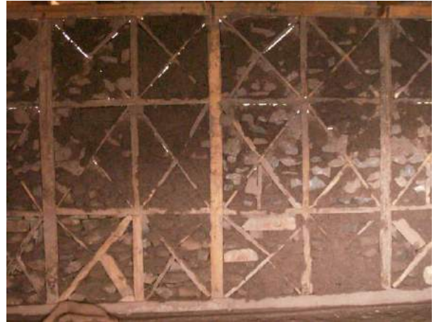
Figure 4a: Thin bracing boards (less than 1" thick) are frequent, but should be avoided
