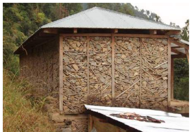
Figure 3g: V-shaped braces with main posts, with or without secondary subdivision
