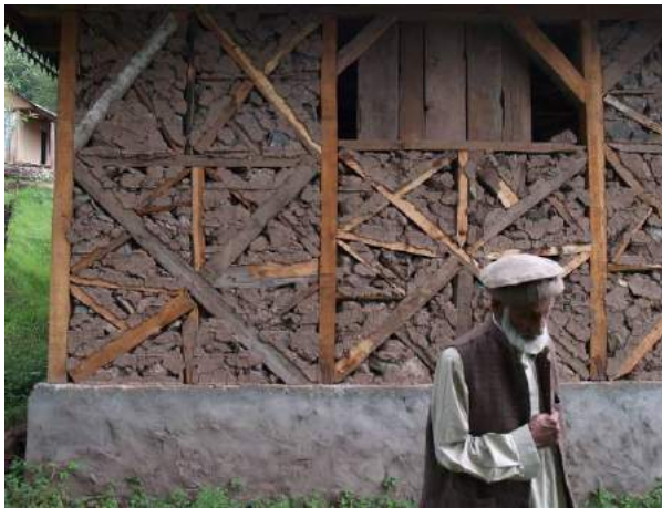
Figure 3h: irregular bracing and use of salvaged timber
