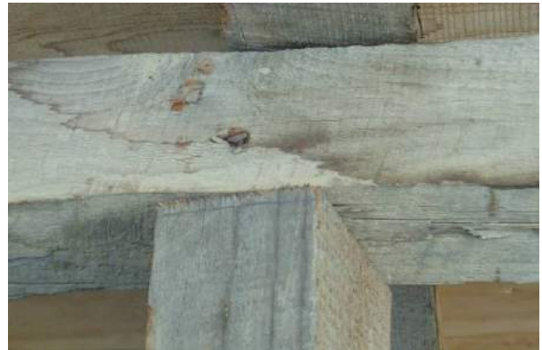
Figure 6e: Fixing through one or two lateral nails
