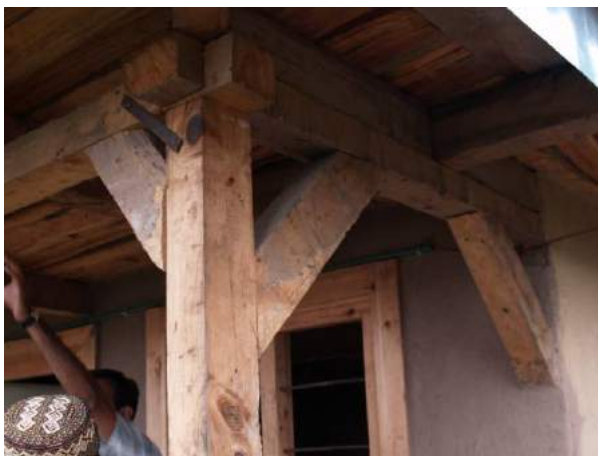
Figure 6g: Rare example of bracings on veranda posts
