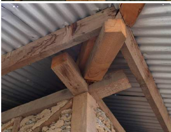
Figure 8k: Same issues at the post – wall plate level. Top: Solution proposed by SDC demonstration model
