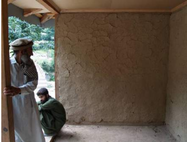
Figure 14a: excessive water in the plaster mixture results in cracks when drying.
