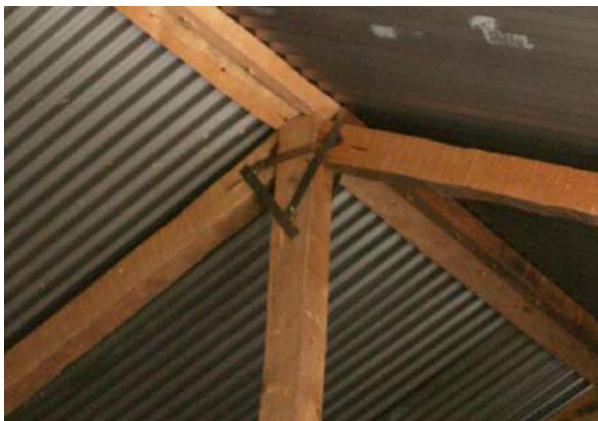
Figure 11k: approximate kingpost on the left, false (standing) kingpost on the right
