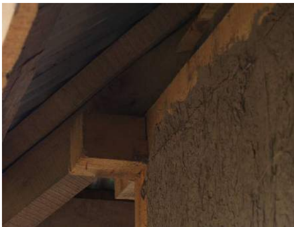
Figure 5b: proper connection and insufficient strength of laps due to insufficiently high wall plates
