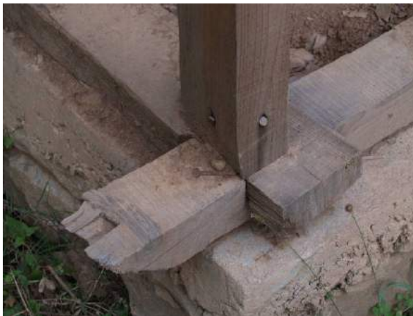
Figure 8a: Nailed connection (four 6" nails)
