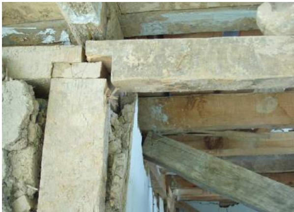
Figures 7c: Short lap joints are insufficient
