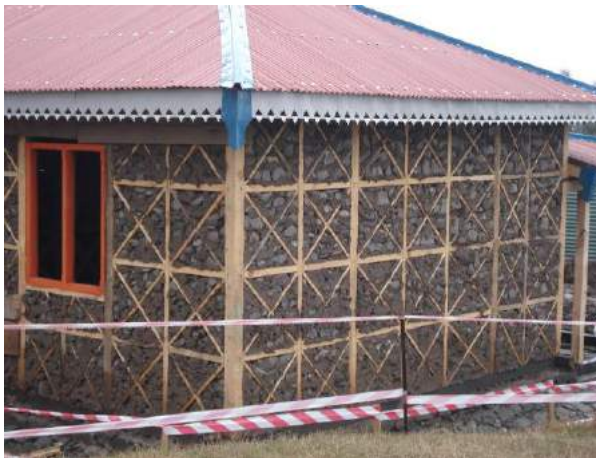
Figure 3a): braced squares pattern, wall height divided into 4 parts
