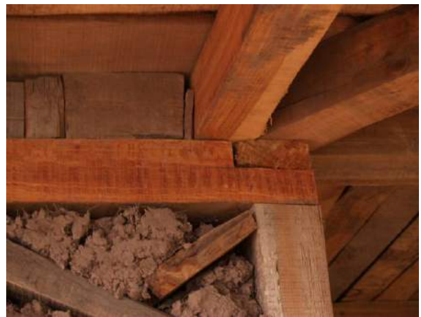
Figure 6f: insufficiently strong corner connection (hold only through vertical nails)
