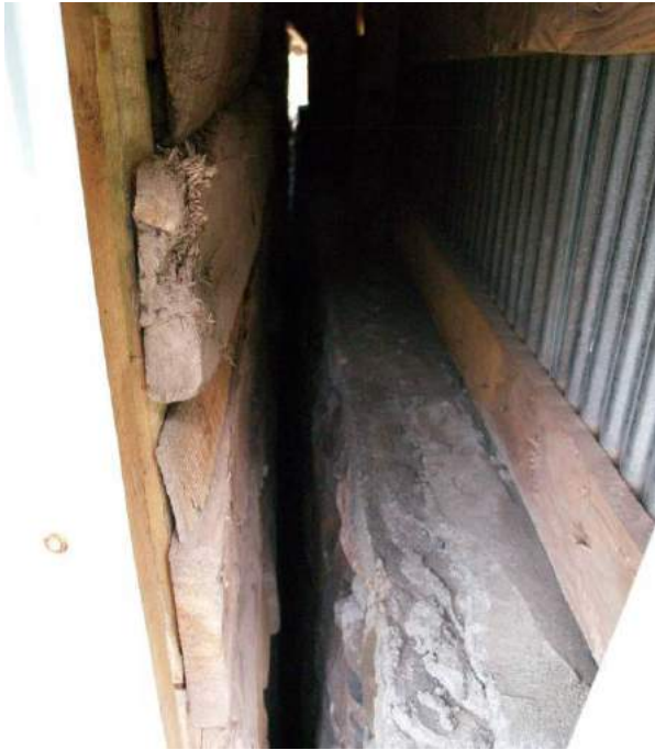
Figure 10a: Dhajji wall very close to retaining wall, void covered by a roof and added wall against snow and rain
