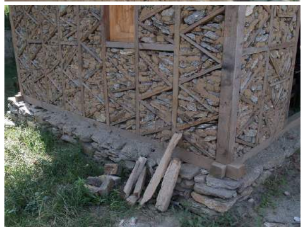
Figure 1c) dry stone masonry without top mortar, leaving room for the water to dry off.
