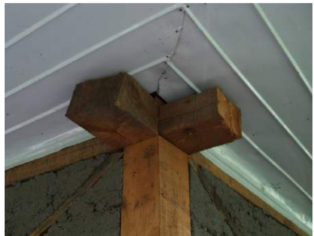
Figure 5b: proper connection and insufficient strength of laps due to insufficiently high wall plates
