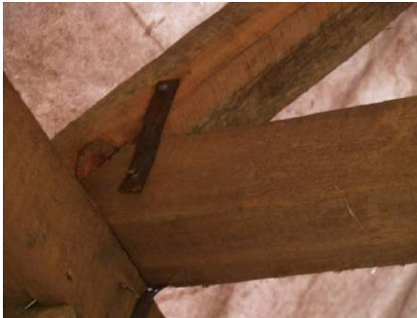
Figure 11f: Correct detail of a tie beam as taught in the trainings.
