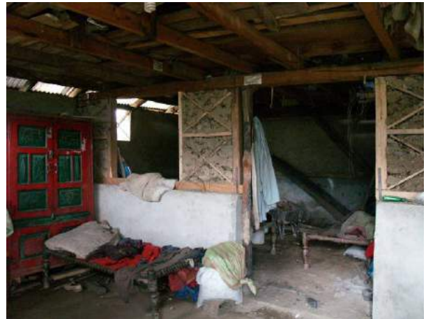
Figure 3e: Braced squares, half height dhajji on half height stone walls (dhajji base plate tied to foundation through stone wall with tie rod).
