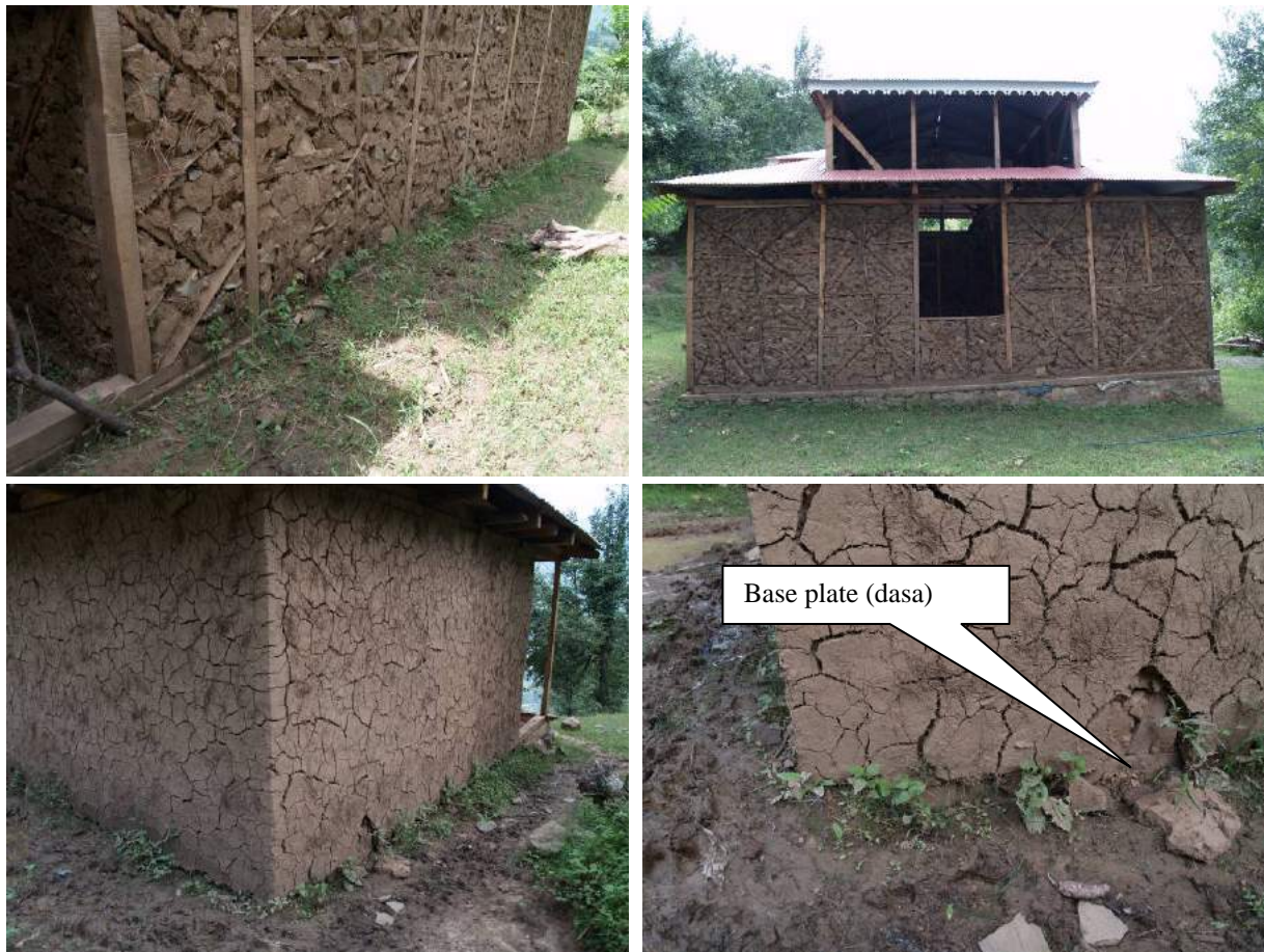
Figure. 1a: Foundations too low and base plate in contact with the ground. Note sufficient height of foundation towards the valley
