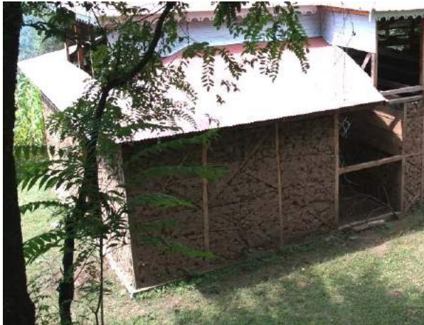
Figure 3d) braced squares, wall height divided into 2 parts. The walls in the lower picture are quite shaky.
