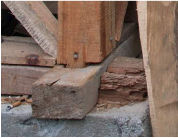
Figure 8b: Mortise and tenon joint. Top left: ERRA poster; Top right: probable joint as per ERRA poster; Lower row: weakening of corner joint through mortise and tenon.
