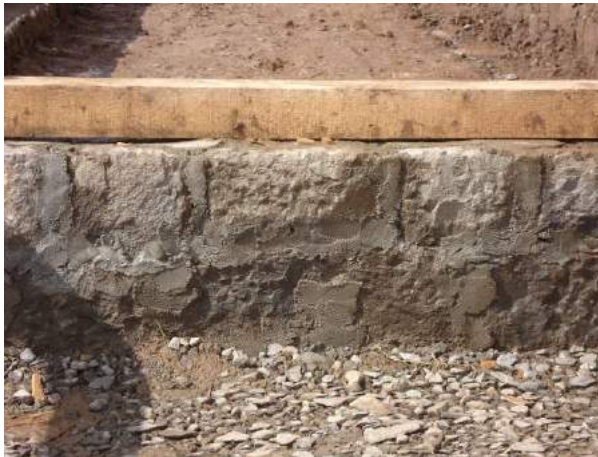
Figure 1b: smooth mortar finish on top of foundation traps water under base plate. Lower left: irregular top surface allowing for water to dry off. Lower right: interesting detail of detaching base plate through spacers
