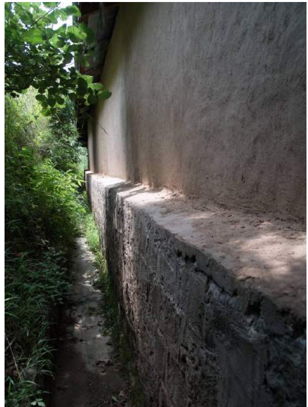
Figure 10g: Back wall in stone masonry, here because a damaged stone masonry house has been transformed in a dhajji house, leaving the lower part of the stone wall.
