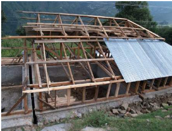
Figure 11i: Rare examples of tie-beams nailed laterally to the rafters
