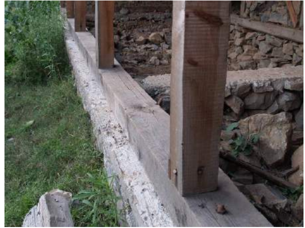
Figure 2a: 99% of new base plates are 4x4", with rare exceptions where salvaged timber is used (right).
