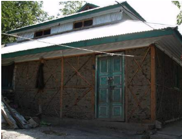
Figure 3c): braced squares, wall height divided into 3 parts in Bhedi (AJK)
