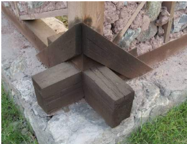
Figure 8f: Corner blocks only on the outside
