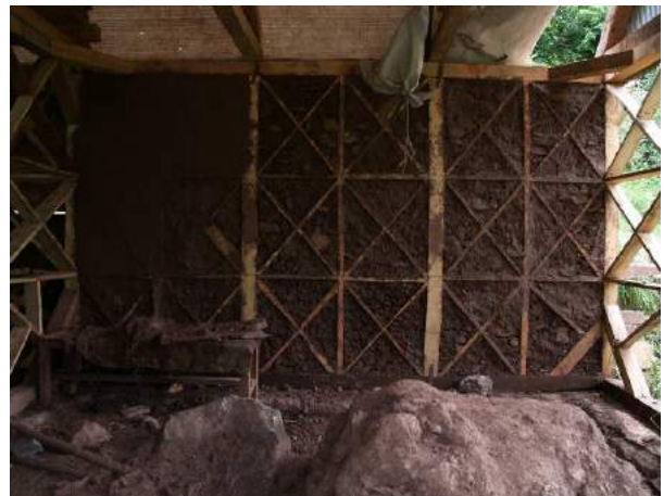
Figure 13a: Infills should mainly be of stones with a limited amount of mud.
