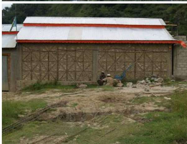
Figure 15a: composite structures concrete - dhajji
