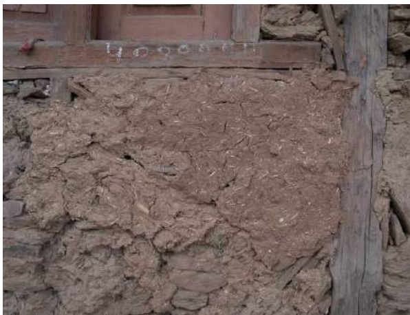
Figure 14c: added straw or pine needles are rarely found (left: pre-EQ building; right: external plaster on a new house)
