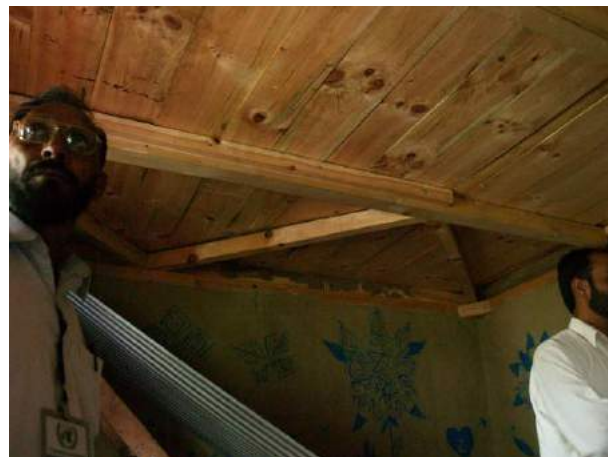
Figure 5d: Horizontal floor bracing
