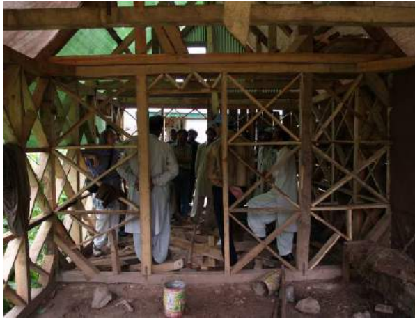
Figure 3c): braced squares, wall height divided into 3 parts in Bhedi (AJK)
