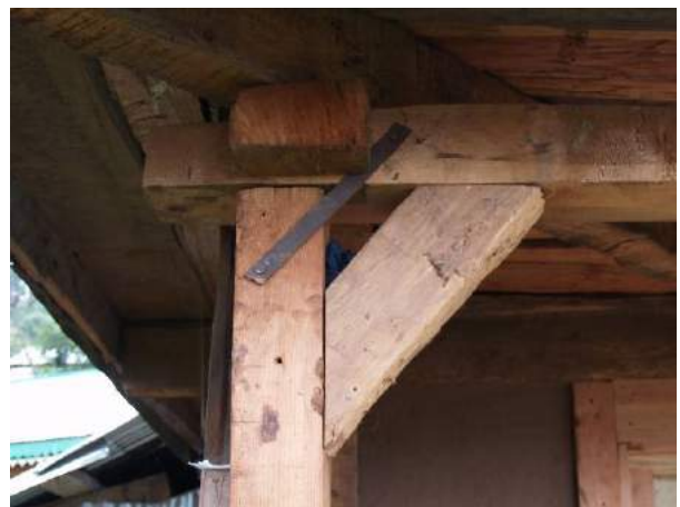
Figure 6f: insufficiently strong corner connection (hold only through vertical nails)
