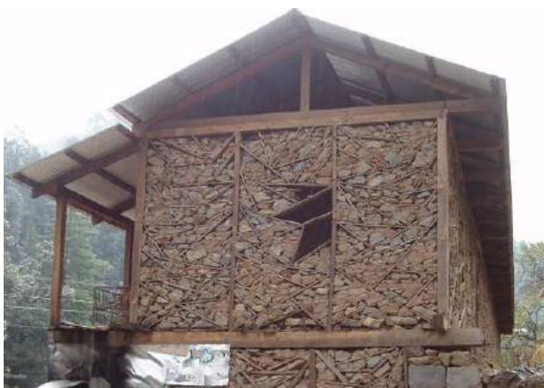
Figure 3g: V-shaped braces with main posts, with or without secondary subdivision
