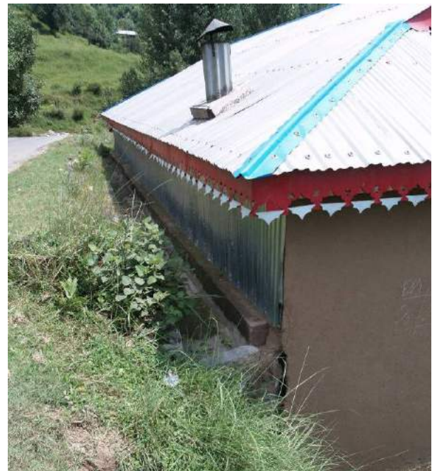
Figure 10c: A dhajji wall against a retaining wall?
