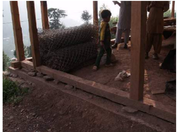
Figure 1b: smooth mortar finish on top of foundation traps water under base plate. Lower left: irregular top surface allowing for water to dry off. Lower right: interesting detail of detaching base plate through spacers
