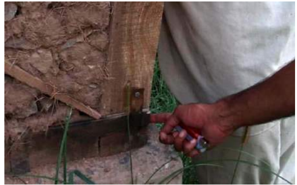
Figure 8b: Mortise and tenon joint. Top left: ERRA poster; Top right: probable joint as per ERRA poster; Lower row: weakening of corner joint through mortise and tenon.
