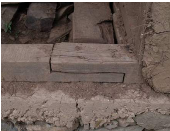
Figure 7b: Long lap joints
