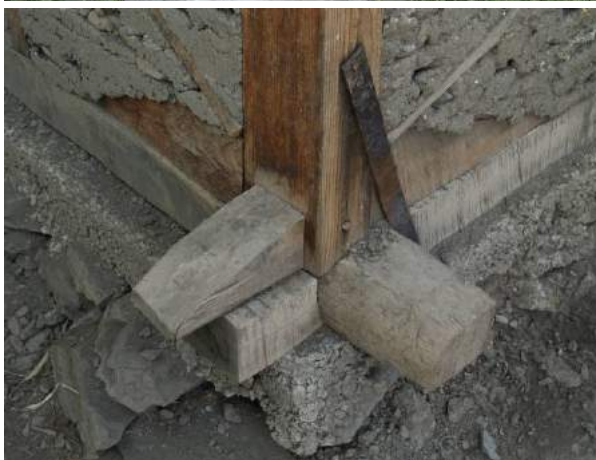
Figure 8g: Joint with inner and outer blocks secured with a diagonal strap (timber board or metal strap)
