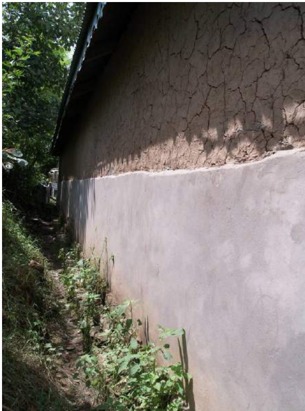
Figure 10g: Back wall in stone masonry, here because a damaged stone masonry house has been transformed in a dhajji house, leaving the lower part of the stone wall.
