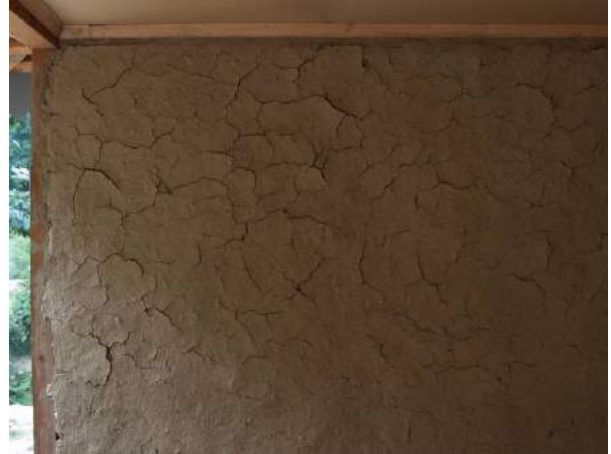
Figure 14a: excessive water in the plaster mixture results in cracks when drying.
