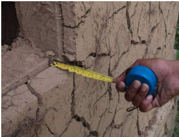
Figure 14b: excessive thickness of a single plaster layer results in cracking.
