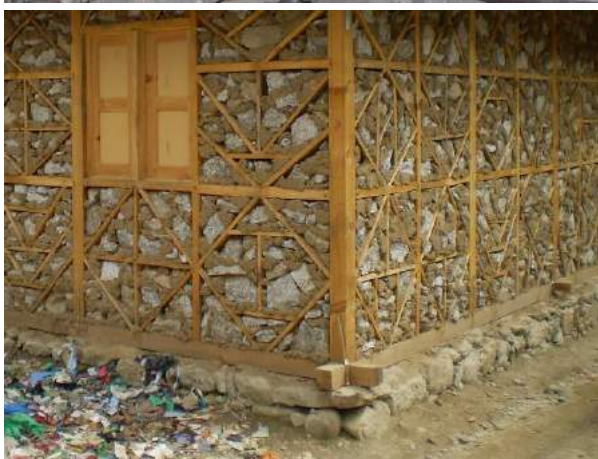
Figure 1c) dry stone masonry without top mortar, leaving room for the water to dry off.
