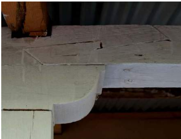
Figure 7a: Interlocking or splayed scarf joints (Kashmiri joints)
