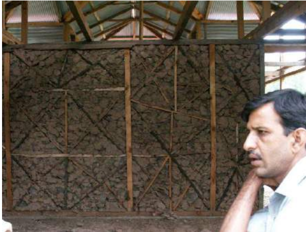
Figure 4a: Thin bracing boards (less than 1" thick) are frequent, but should be avoided
