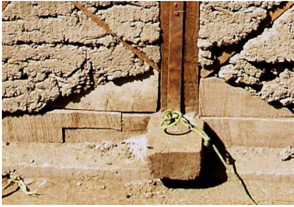
Figure 6c: lateral blocks as suggested by ERRA
