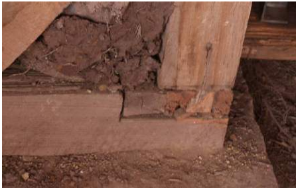
Figure 8c: cut off ends of dasa weakening the corner, even with a strap.
