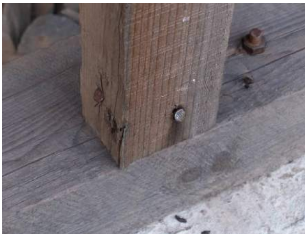
Figure 6a: Most joint are simply nailed, mostly with four 6" nails
