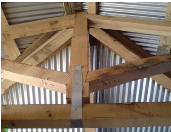
Figure 11j: Proper (hanging) kingposts have only been observed once.
