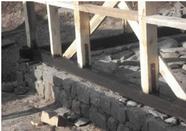
Figure 2b: base plate treatment with old engine oil;
