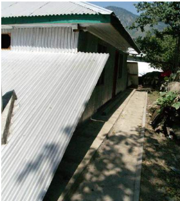
Figure 10b: backside of second storey, ground floor against retaining wall. Ground floor back wall identical with retaining wall?
