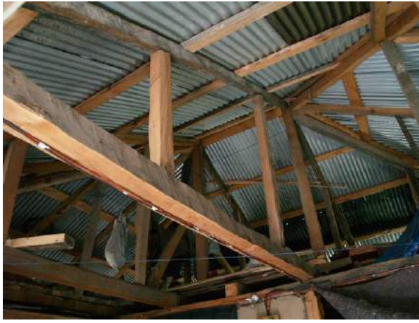
Figure 11 l: typical roof structures with standing posts
