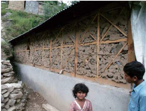
Figure 3e: Braced squares, half height dhajji on half height stone walls (dhajji base plate tied to foundation through stone wall with tie rod).
