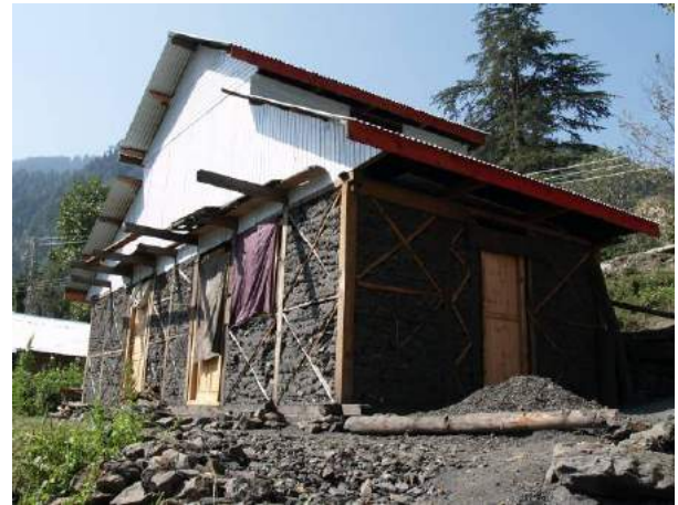
Figure 3c): braced squares, wall height divided into 3 parts in Bhedi (AJK)
