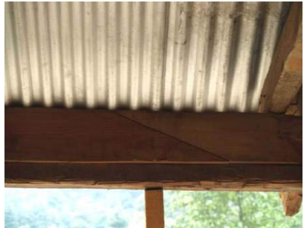
Figure 7e: Simple scarf joint
