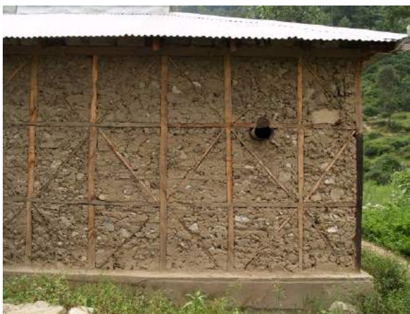
Figure 3b: examples of 'half-braced' small squares
