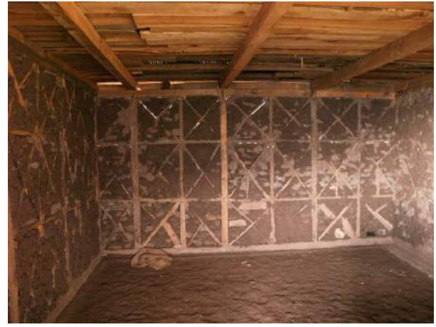
Figure 3c): braced squares, wall height divided into 3 parts in Bhedi (AJK)
