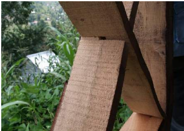
Figure 4b: lapped bracings: good or bad?
