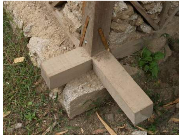
Figure 8j: simple straps in addition to nails might not be strong enough (to be tested)
