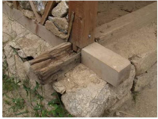
Figure 8b: Mortise and tenon joint. Top left: ERRA poster; Top right: probable joint as per ERRA poster; Lower row: weakening of corner joint through mortise and tenon.
