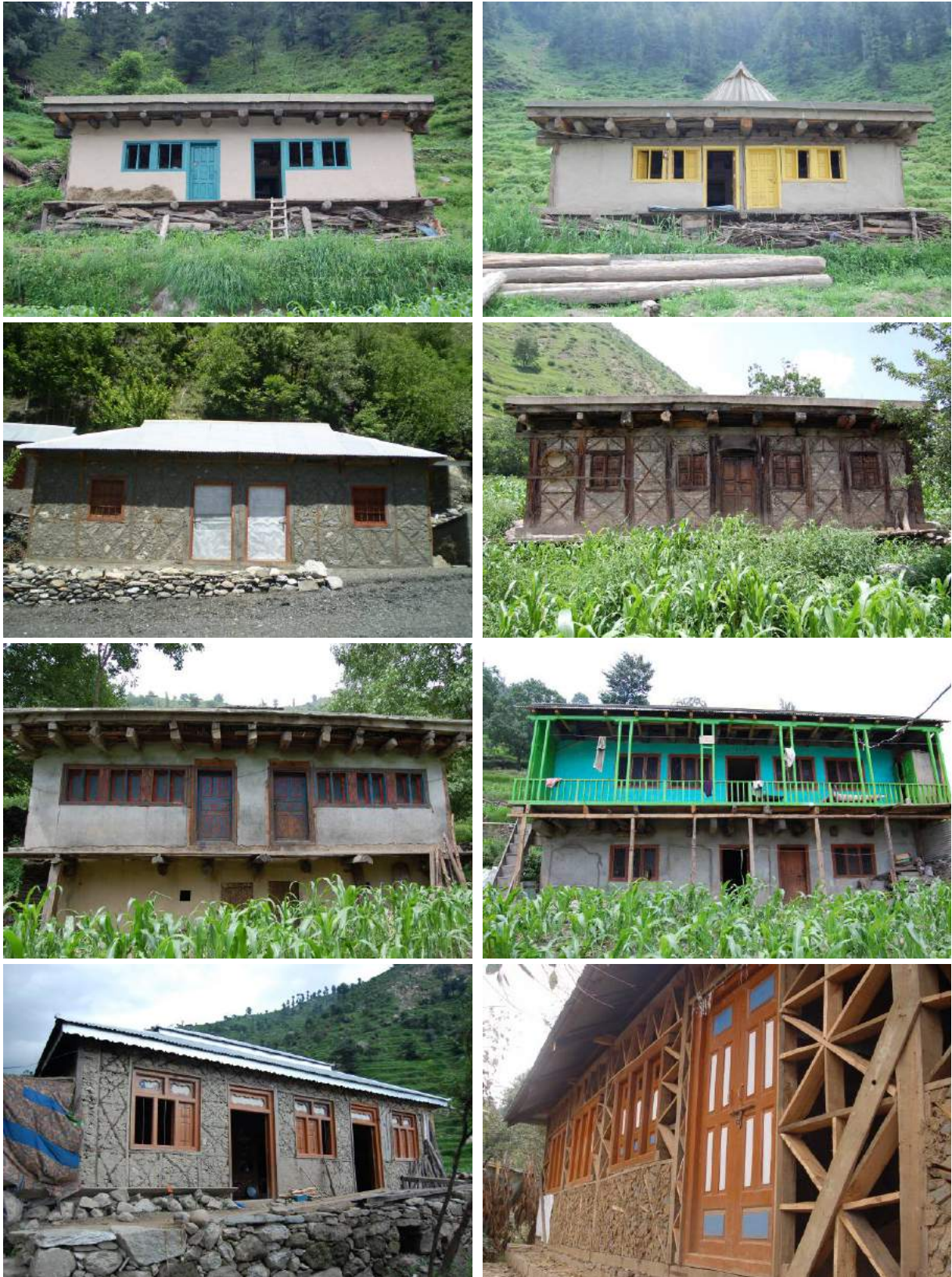
Figure 12a: High number of openings on the front side, which can become problematic.
