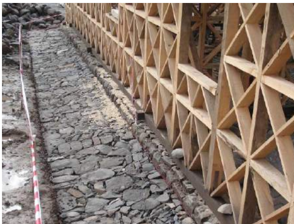
Figure 2c: Passive protection through run off skirt
