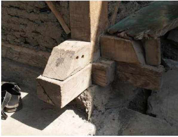
Figure 8f: Corner blocks only on the outside
