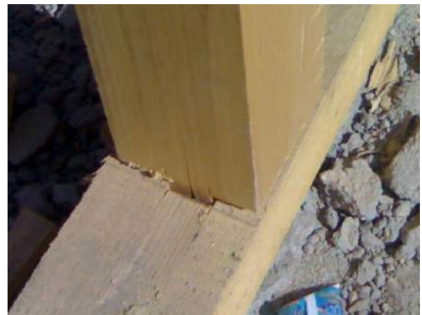
Figure 6b: Mortise and tenon joint
