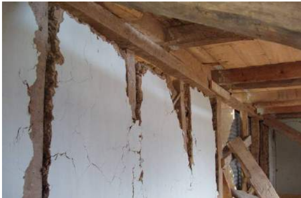
Figure 6d: Insufficient number of nails and nails too short (example after earthquake)
