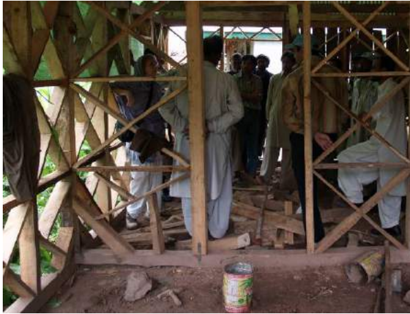
Figure 2a: 99% of new base plates are 4x4", with rare exceptions where salvaged timber is used (right).
