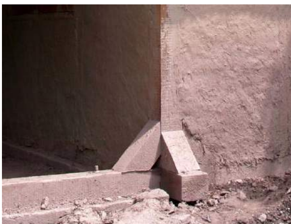
Figure 8e: Corner blocks inside and outside of the post.
