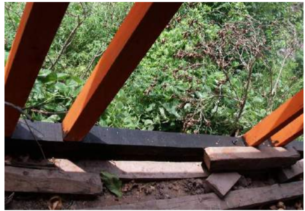
Figure 2a: 99% of new base plates are 4x4", with rare exceptions where salvaged timber is used (right).
