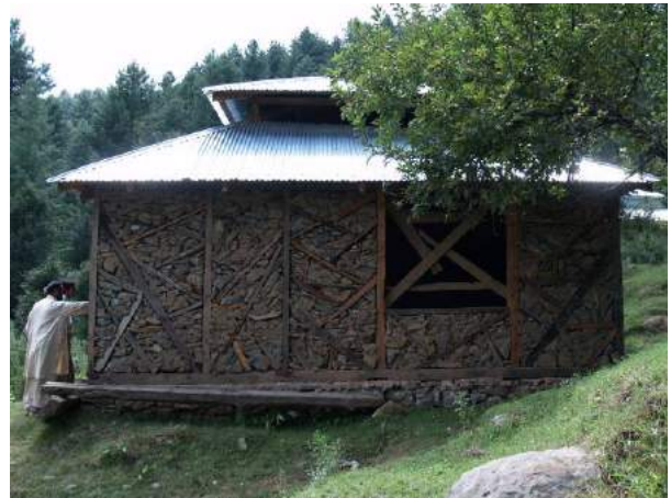
Figure 4c: Irregular fill-in with long corner braces, creating an imbalance.
