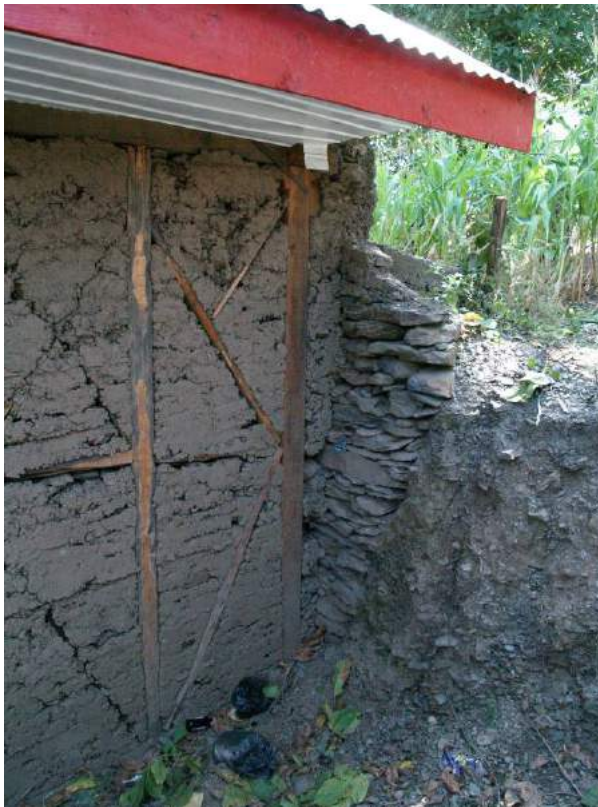
Figure 10e: Dhajji back wall against retaining wall. The upper part of the dhajji wall has been kept without races to allow for storage (i.e. weak dhajji wall).
