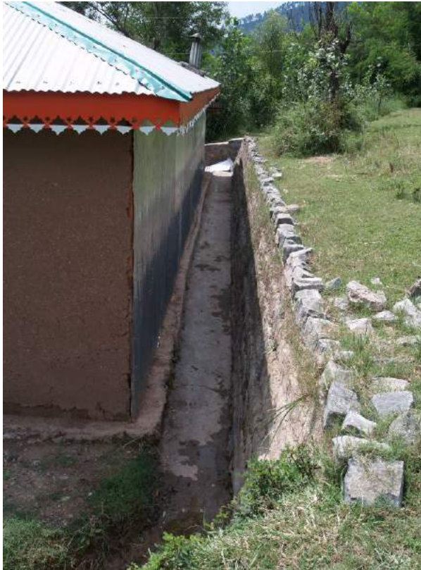
Figure 10f: a well done channel between a retaining wall and a dhajji back wall
