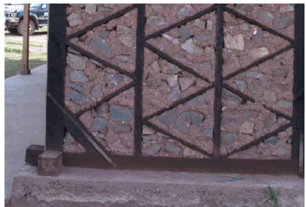
Figure 8i: Short corner braces: a good thing or causing an dangerous lever that adds more strain to the corner?
