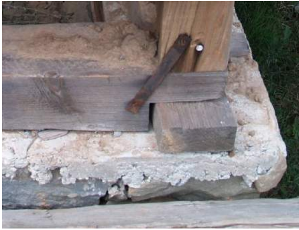
Figure 8j: simple straps in addition to nails might not be strong enough (to be tested)
