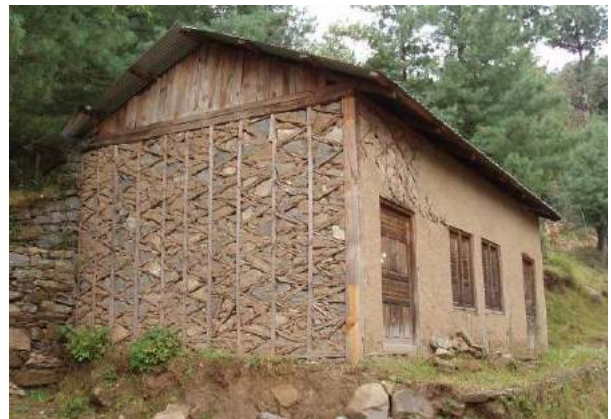
Figure 3e: Braced squares, half height dhajji on half height stone walls (dhajji base plate tied to foundation through stone wall with tie rod).
