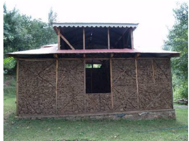
Figure 3d) braced squares, wall height divided into 2 parts. The walls in the lower picture are quite shaky.
