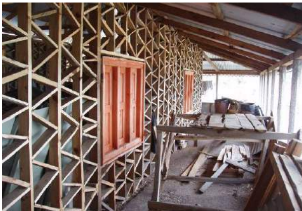
Figure 3f: Zig-zag braces and close spacing of vertical posts (boards)
