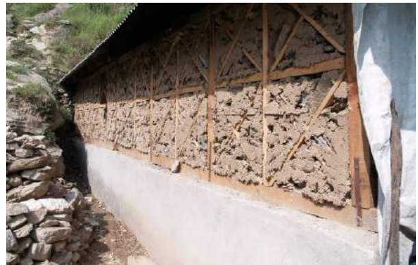
Figure 10d: Lower part stone masonry, upper part dhajji, against a retaining wall, all covered by a concrete slab.
