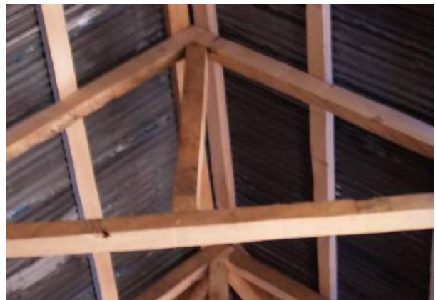
Figure 11k: approximate kingpost on the left, false (standing) kingpost on the right
