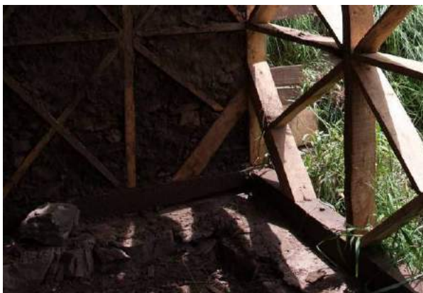
Figure 8i: Short corner braces: a good thing or causing an dangerous lever that adds more strain to the corner?
