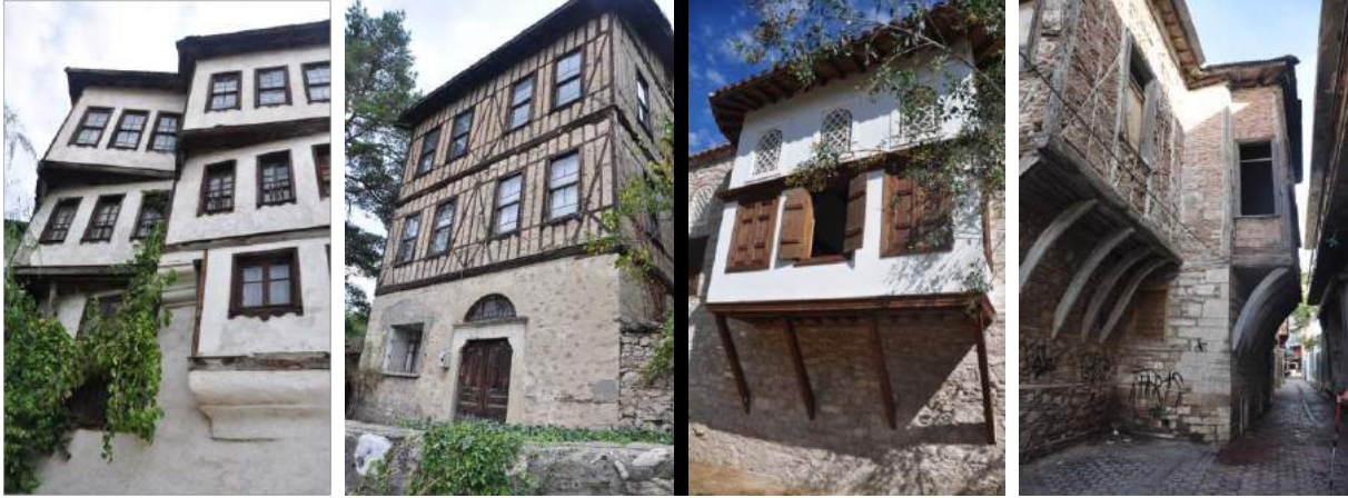
Figure 1. Examples to himiř houses in Turkey (first two photos, Safranbolu) and in Greece (last two photos, Athens and Chalkis, respectively)
