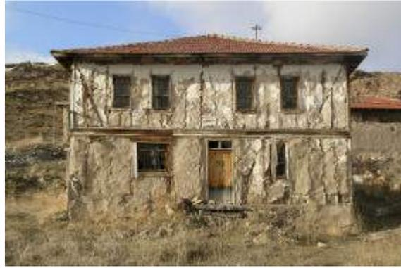
Figure 3.3. 'Himis' structure with sun-dried brick infill from Central Anatolia
