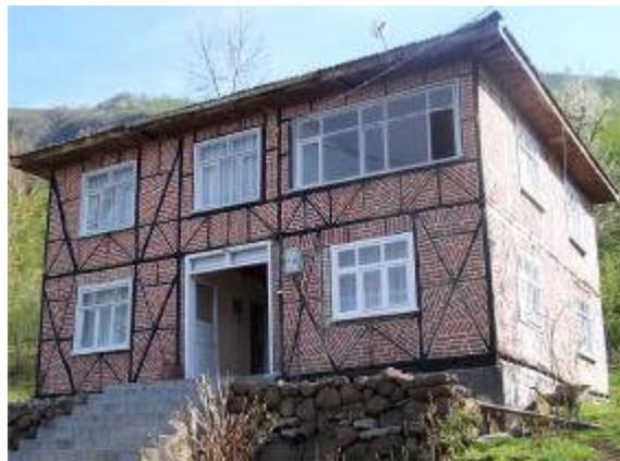
Figure 3.4. 'Himis' structure with brick infill from Western Black Sea region
