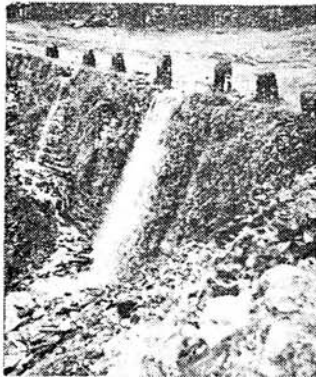
PHOTO 8. Toe wall at bottom dissipates the energy of falling rain water and avoids toe erosion
