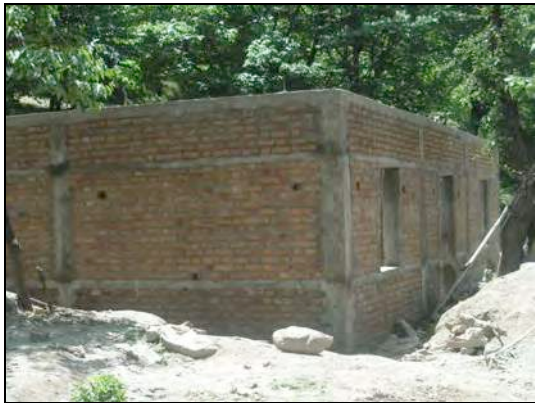
Fig. 3: Seismic bands at sill and lintel level
