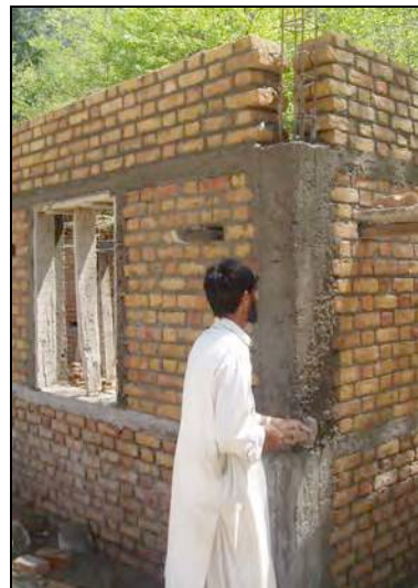
Fig. 6: Pouring concrete bit by bit
