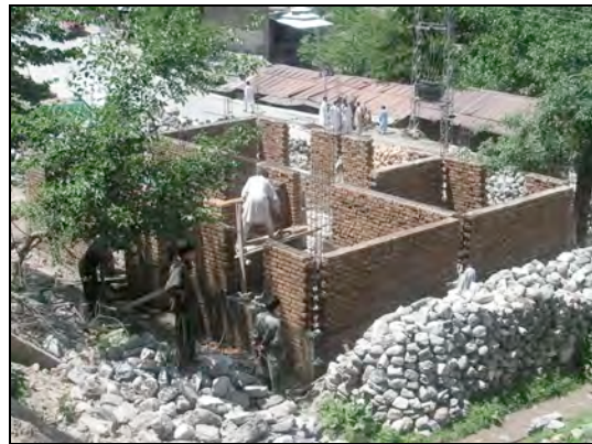
Fig. 4: Raising wall from sill to lintel band before pouring of the tie-columns
