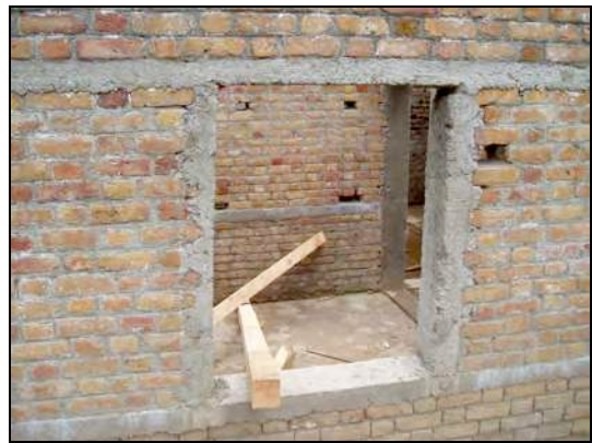
Fig. 12: Vertical bands around openings
