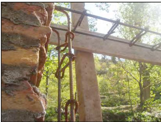
Fig. 11: Vertical band around openings
