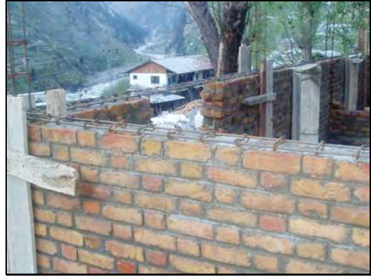
Fig. 8: Seismic band at lintel level
