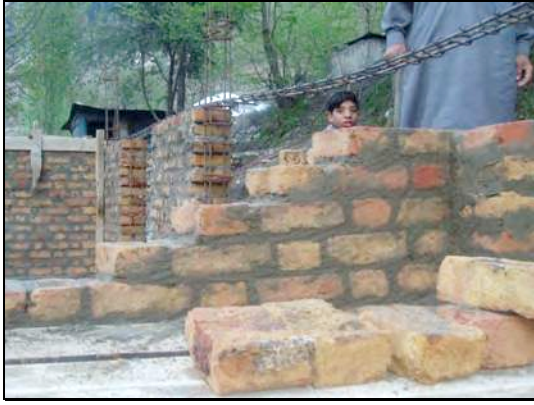
Fig. 7: Seismic band at lintel level
