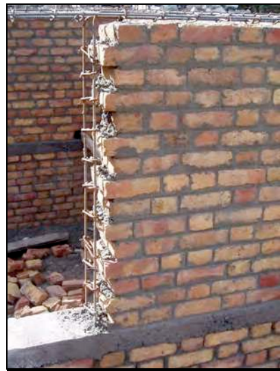
Fig. 10: Vertical reinforcements around openings
