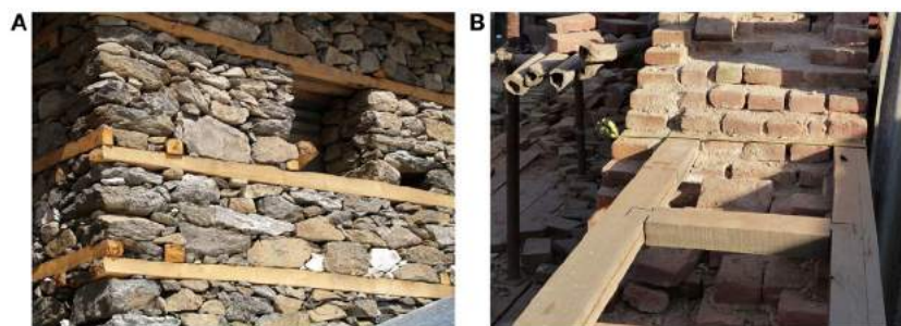
FIGURE 1 | (A) Wooden bands and dry-stacked rubble stone masonry (photo credit: Tom Schacher). (B) Wooden bands and brick masonry with lime mortar in Bhaktapur, Nepal (photo credit: Martijn Schildkamp).
