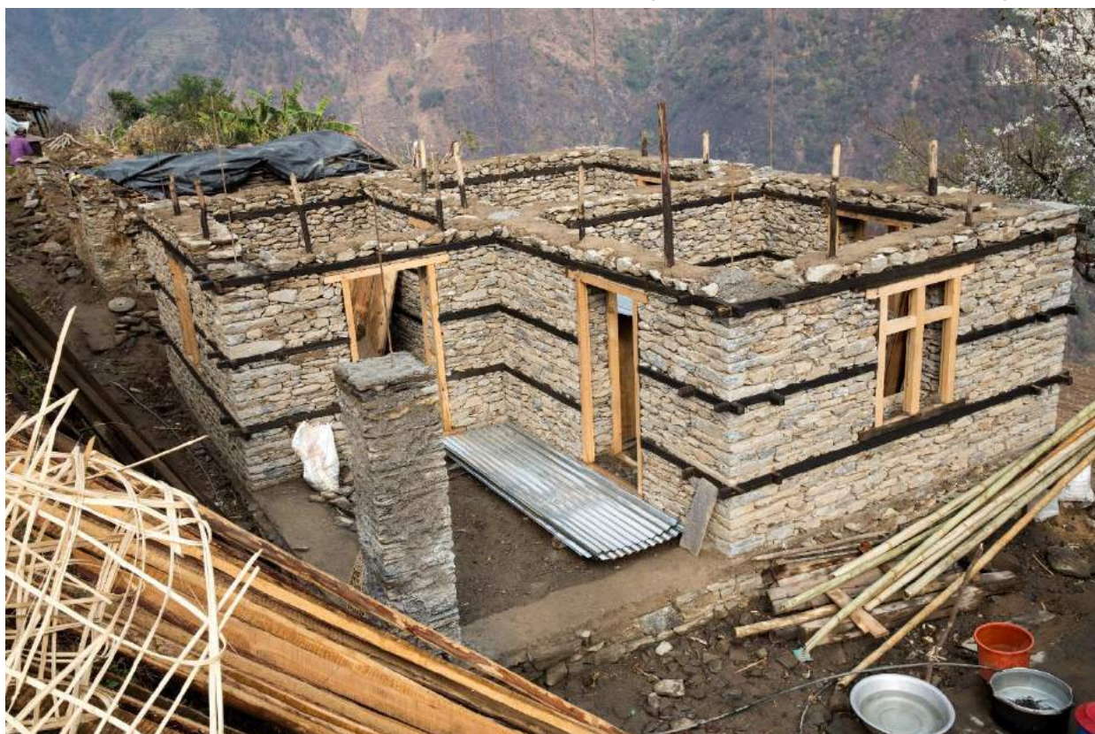
Mitra Tamang's new house is almost finished!
