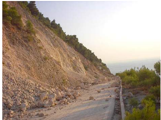
Fig. 4. Road connecting villages of Tsoukalades and Kathisma cut off by landslides (courtesy: A. Anastasiadis, Dpt. of Soil Dynamics, ITSAK).
