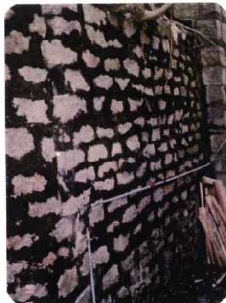
Plate B10 - Tied Face Wall with Horizontal Beams (11SW-A/R45)
