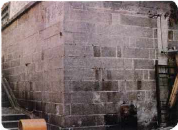
Plate B9 - Tied Face Wall (11SW-A/R74)
