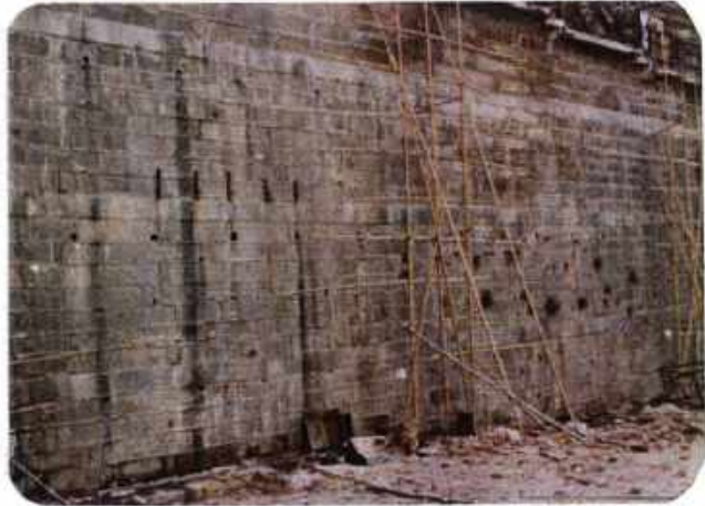
Plate B10 - Tied Face Wall with Horizontal Beams (11SW-A/R45)
