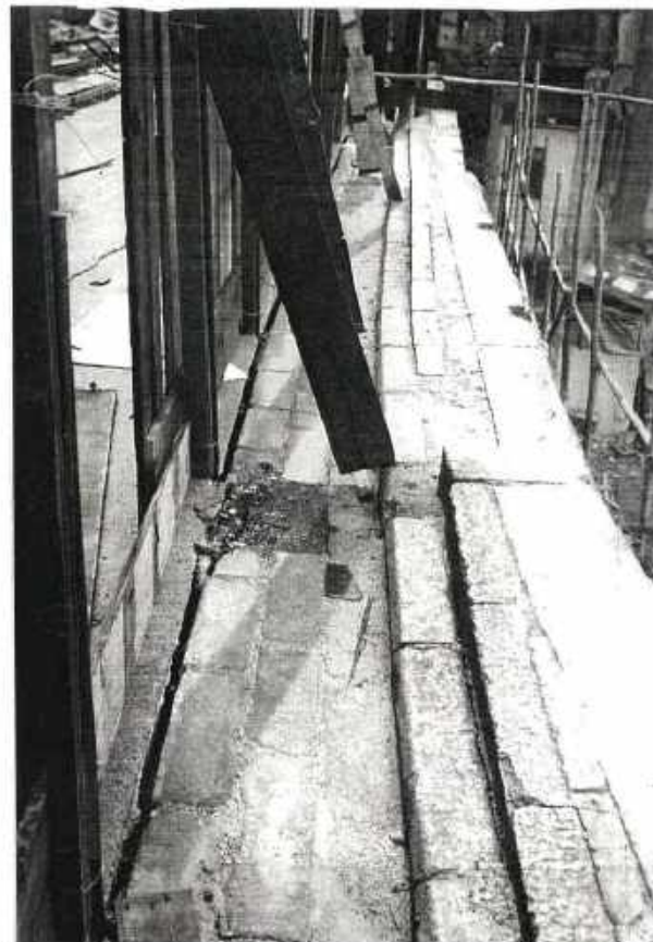
Plate D6.11 - Retaining Wall at Circular Pathway - Detail of the Cracks on the Pathway (I)
