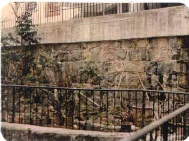
Plate B5 - Pointed Squared Rubble Wall (11SW-A/R295)
