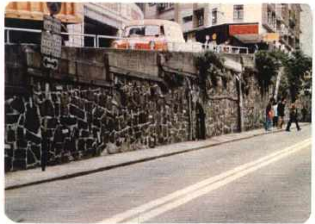
Plate B2 - Pointed Random Rubble Wall (11SW-A/R116)
