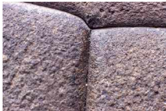
Fig. 7. These joints of stones from Inca walls in Cuzco clearly show, that in their neighbourhood the surface properties of the stone material is different in colour and structural composition from the rest of the stone material.
