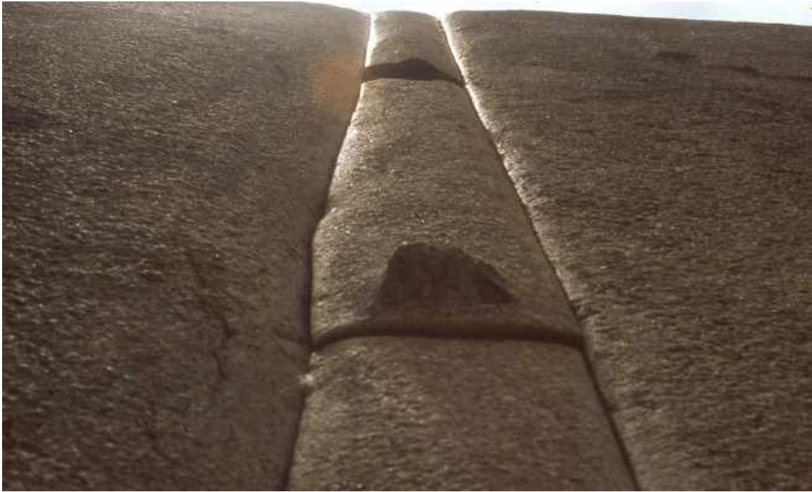
Fig. 6. When looking up the nearly 4 m long stone joints between the standing stone blocks of the Wall of the six Monoliths in Ollantaytambo one recognizes, that only these joints seem to have received a special treatment, which is generating a high light reflection.
