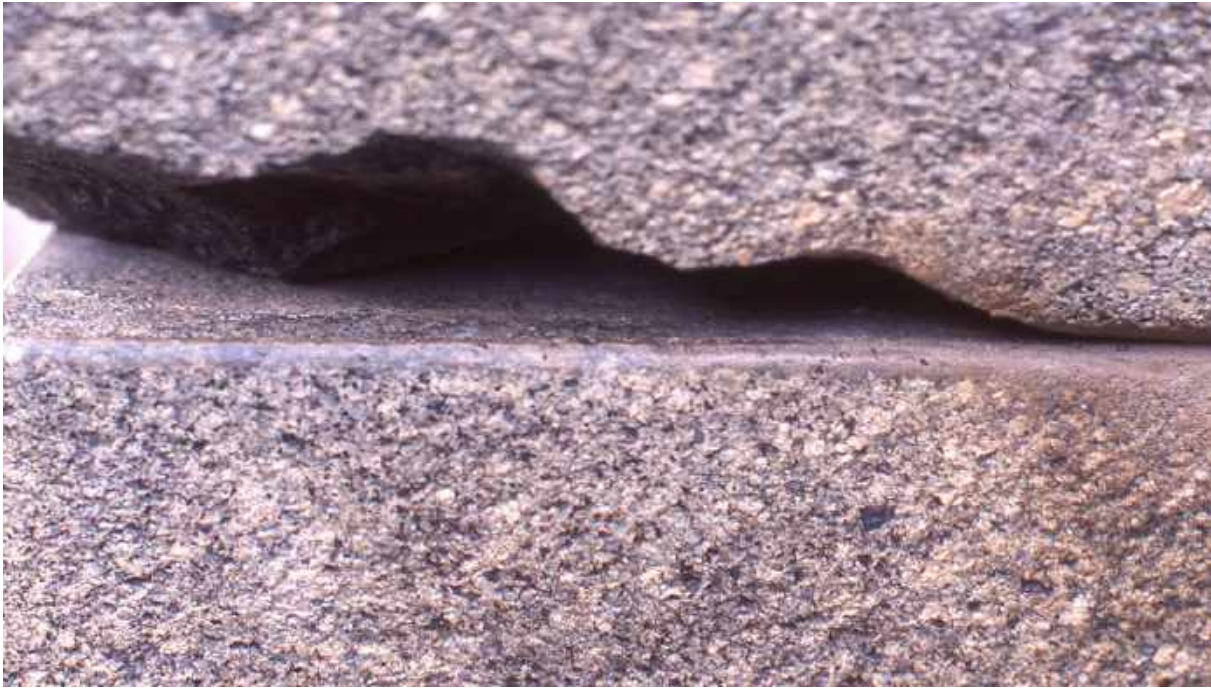
Fig. 8. In this stone junction from Sacsayhuaman (compare fig. 2) part of upper stone is missing and this gives visual access to the surface of the original stone junction, which is much more elaborate and shiny, compared to the rest of the stone surfaces, which were hammered or maybe also polished.
