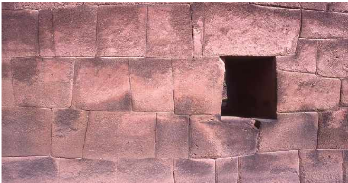
Fig. 4. This wall from the Pisac ruins gives a good impression of the apparent easiness and elegance, with which Inca stone blocks appear to have been laid down. They seem to have been soft, adjusting and settling themselves to perfect fitting via their weight.
