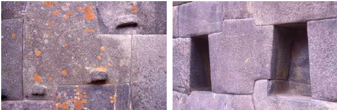
Fig. 3. Tightly fitted Rhyolite boulders in Inca walls at Ollantaytambo, additionally showing a characteristic uneven surface shape. The process of cutting them from solid volcanic rock and shaping them to such perfection with stone hammers and grinding movements, as presently explained, remains an admirable achievement.
