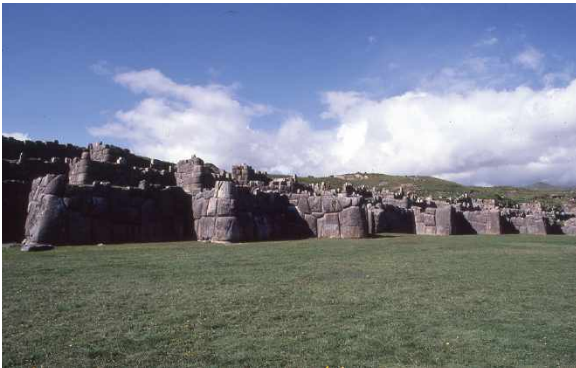
Fig. 2. The Sacsayhuaman fortress near Cusco became a symbol of power, expressed through impressive arrangements of huge fitted stone blocks. Polygonal stones show often convex faces and sunken joints providing attractive patterns in sunlight.
