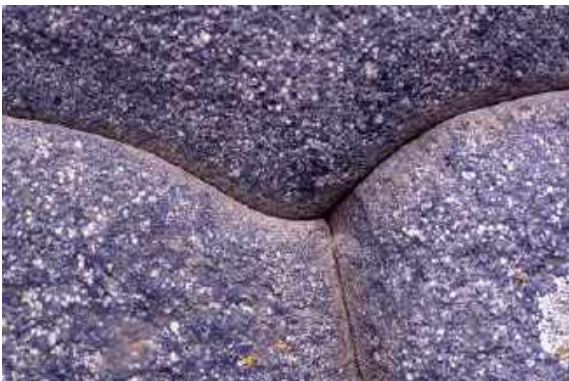
Fig. 7. These joints of stones from Inca walls in Cuzco clearly show, that in their neighbourhood the surface properties of the stone material is different in colour and structural composition from the rest of the stone material.
