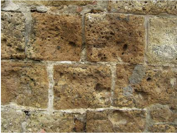
Figure 11.6 Tuff masonry in Pitigliano (Tuscany, Italy).
