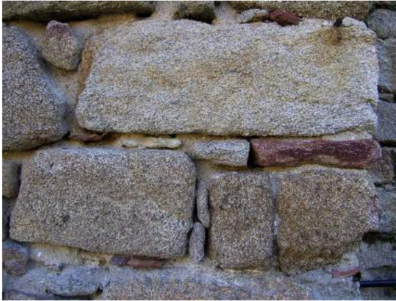
Figure 11.1 Granite ashlars in a building of Giglio island (Tuscany, Italy). Photograph: F. Fratini.
