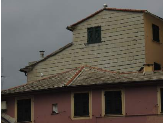
Figure 11.8 The Ligurian slate (ardesia) used as tiles for roofs and wall protection (Genoa, Italy).
