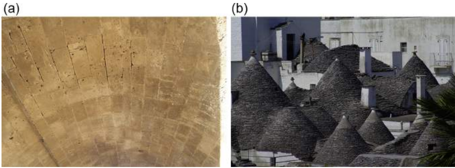
Figure 11.17 (a) Ashlar masonry used in a barrel vault in Ragusa (Sicily, Italy). (Photograph: L. Dipasquale.) (b) Corbelled domes in Alberobello (Apulia, Italy) (Photograph: L. Dipasquale.)
