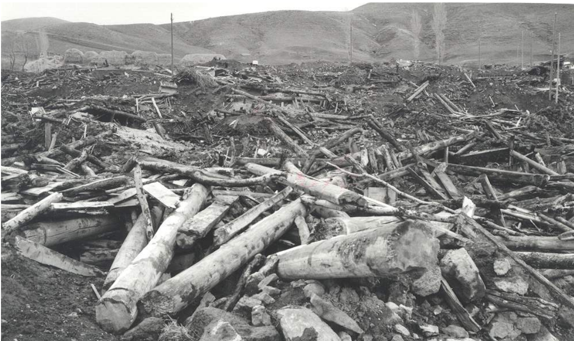
Photograph 1: Erzurum Earthquake Epicentral Damage
