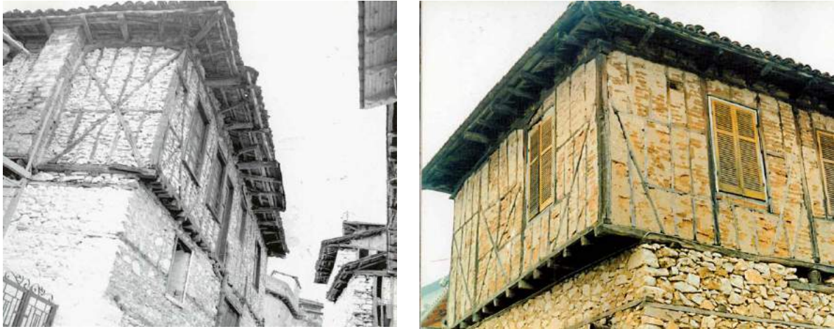
Figure 1. Old traditional buildings with load bearing walls made by "tsatmades"
