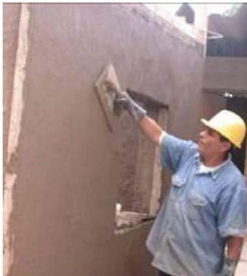
**Figure 14.** Placing the second plaster layer.
