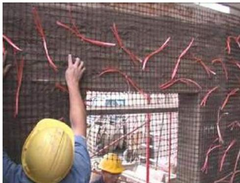
**Figure 9.** Placing and tying the piece of geogrid.
