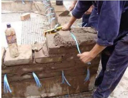
**Figure 7.** Placing plastic strips.
