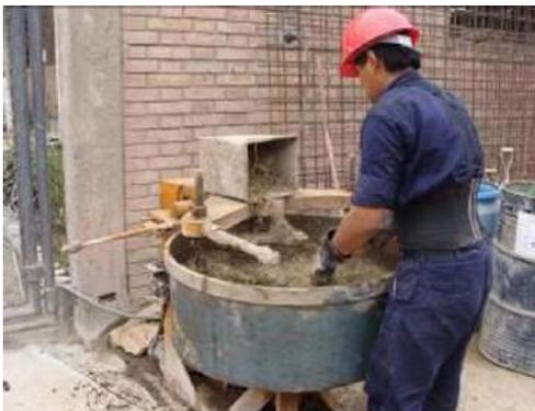
**Figure 12.** Preparing the mortar.
