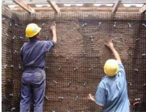
**Figure 13.** Placing the first mud plaster layer.
