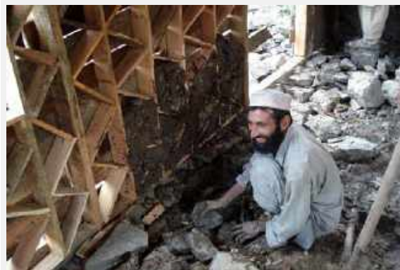
Figure 1. Typical Dhajji Construction in Northern areas of Pakistan
