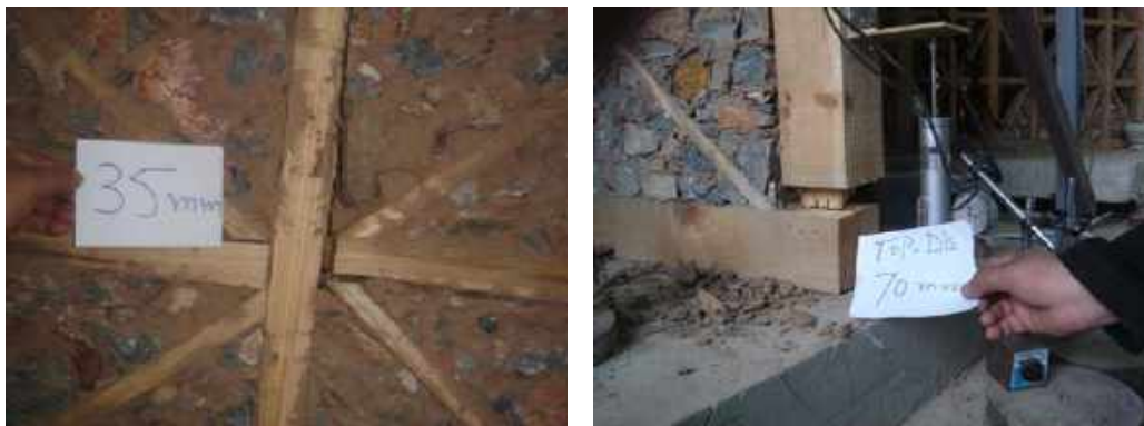
Figure 4. Separation of infill from wooden frame and opening of connections
