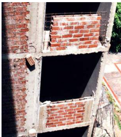
Figure 7. Independent parapets.
