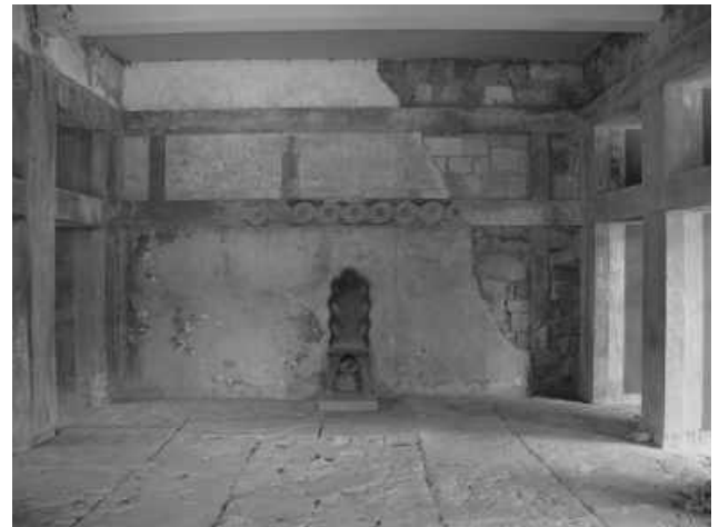
Figure 4. Timber frames of doors in the restored double axes hall of the palace of Knossos (Tsakanika, 2006)
