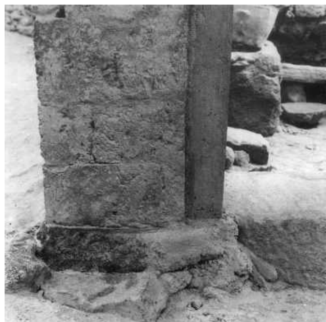
Figure 7. Section D, room D15, northwest exterior corner. The foundation of cut stones (Palyvou, 1999)
