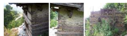
Figure 17. Modification of the Koti Banal construction principle: wooden logs are only arranged as ring beams between layers of stone. The interspacing heights between the layers of wooden logs range between tens of centimeters up to one meter.
