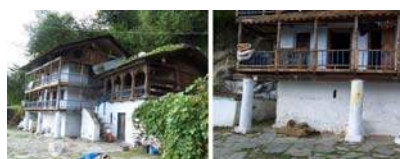
Figure 16. Modification of the Koti Banal construction principle: arrangement of external verandas resting on massive columns.
