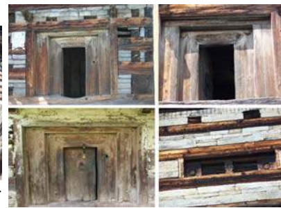
Figure 14. Detailing of door and window openings.
