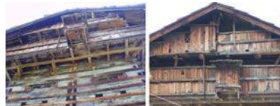
Figure 20. Toilet (outhouse) attached to the balcony at fourth floor at the buildings backside.
