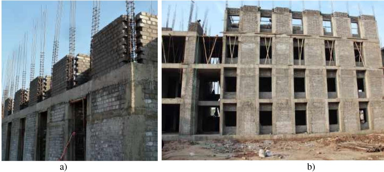
Figure 3: Building construction in progress: a) faculty and staff housing, and b) a hostel.
