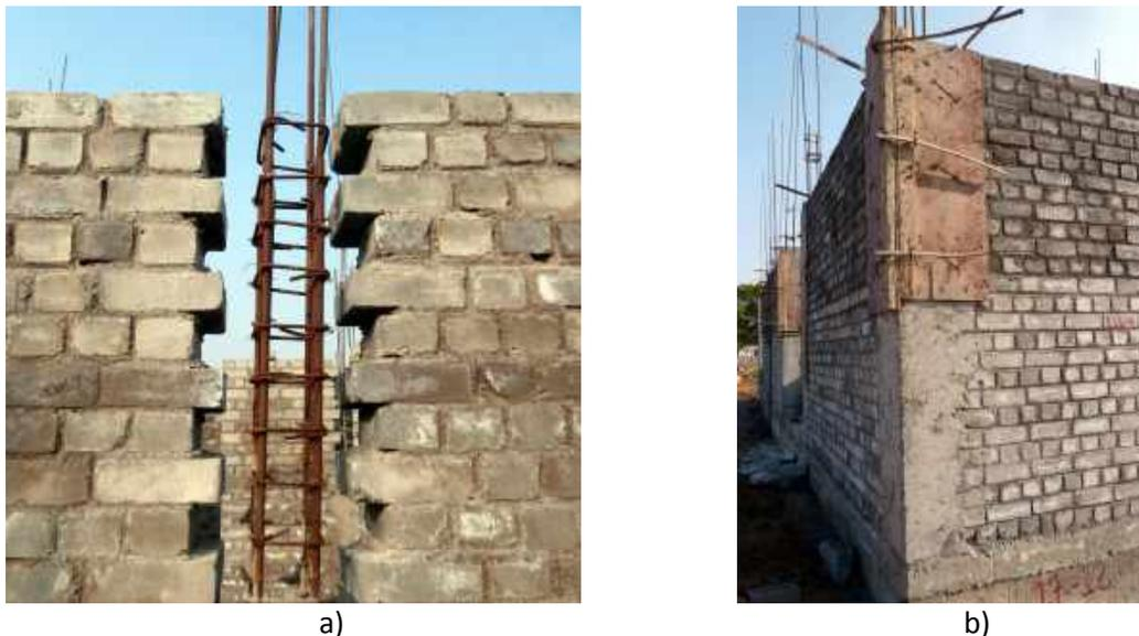
Figure 2: Construction details: a) toothing, and b) formwork for RC tie-columns.
