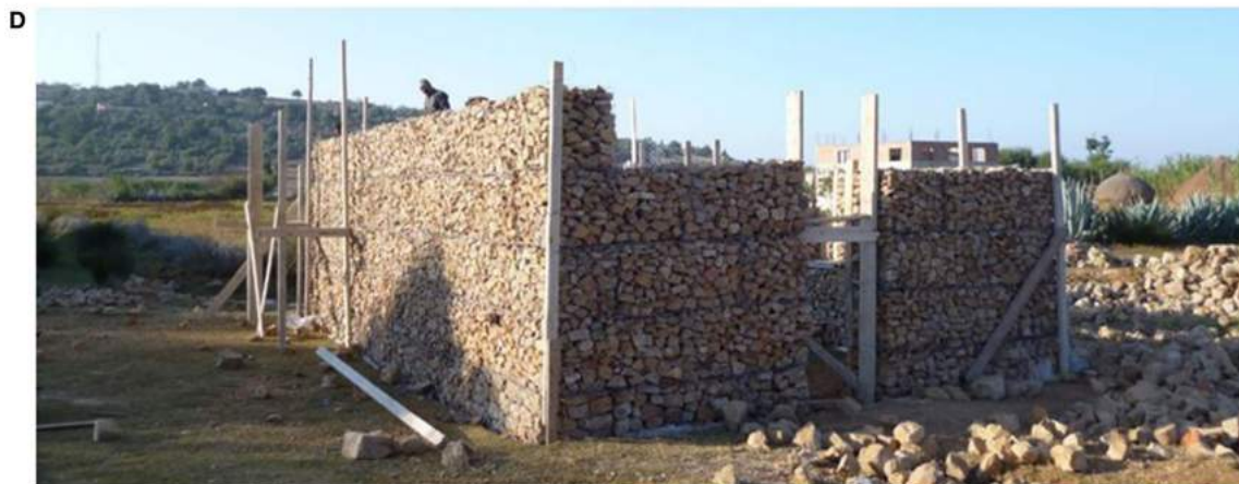
FIGURE 2 | (A) The typical wire mesh. (B) The gabion-box. (C) The gabion-box wall (courtesy from Anping Xingmao Metal Wire Mesh Co., Ltd. ). (D) The gabion-box walls building (courtesy from A&D—Architecture and Development—www.archidev.com working with architecture sans frontières Nepal ).
