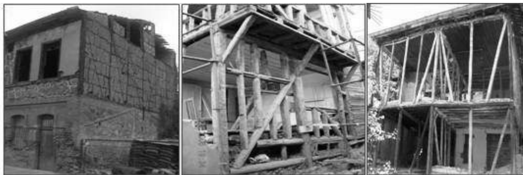
Figure 11. Wooden bearing system and its overhangs.
