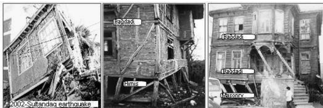
Figure 7. Earthquake damage at soft stories (Dogan 2007)
