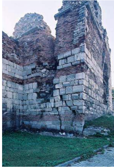
Figure 5 & 6: Istanbul City walls showing brick banding in surviving historic section and collapsed reconstructed section with fake banding.
