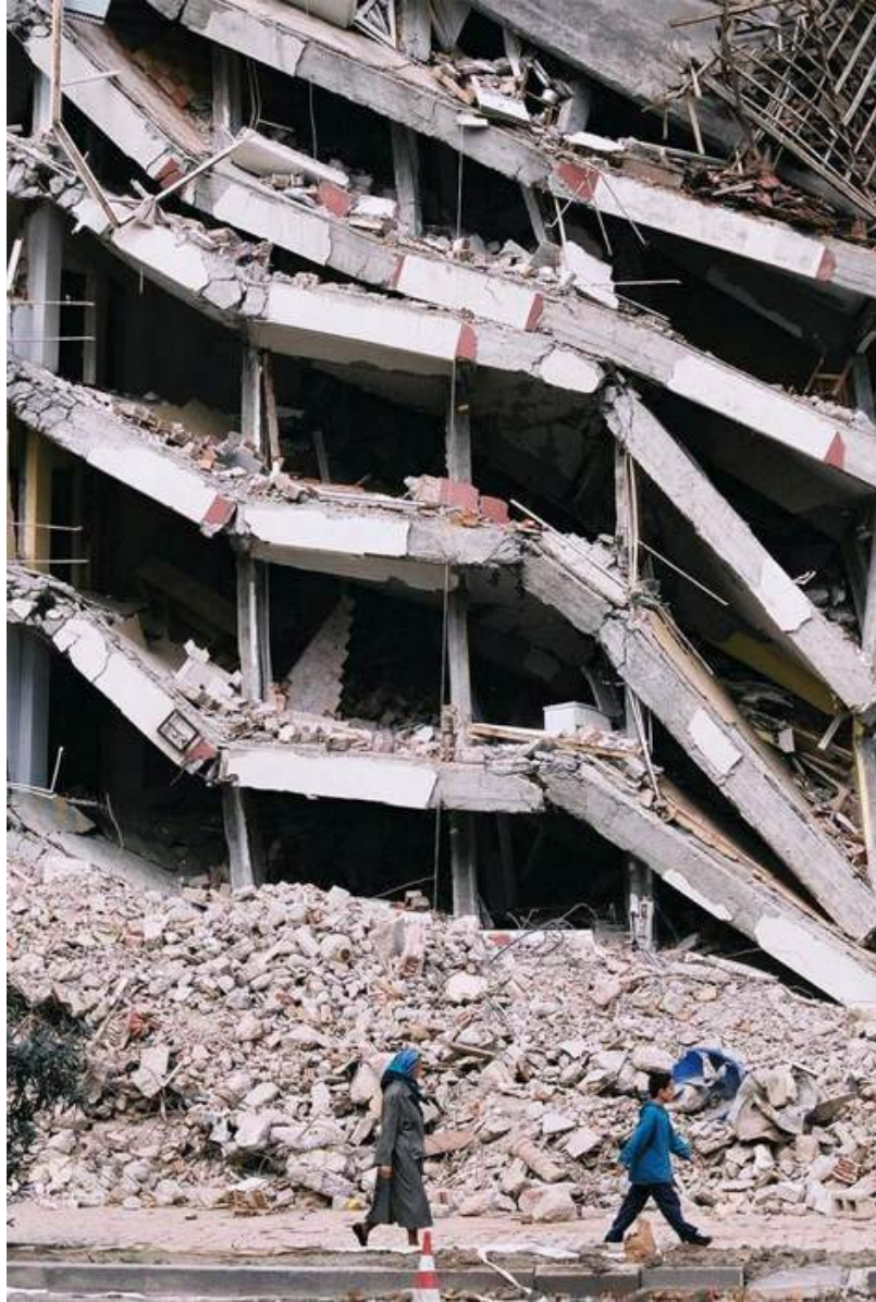
Figure 15: Collapsed Reinforced concrete building in Gölcük.
