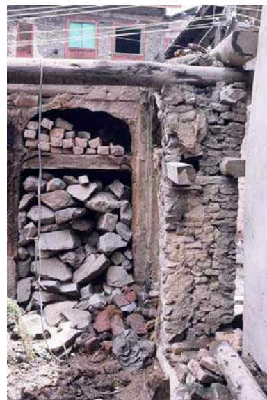
Figure 7 & 8: Taq construction in Srinagar, Kashmir and demolished section of wall showing timber lacing in wall section.
