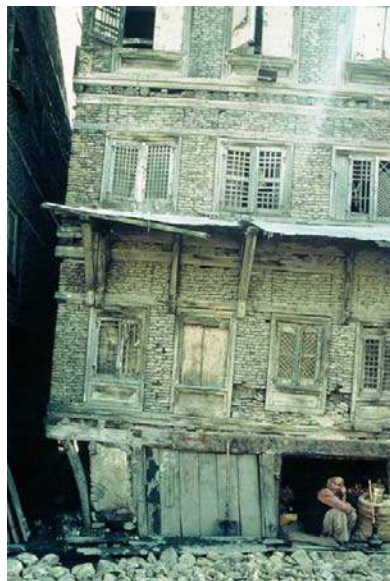
Figure 7 & 8: Taq construction in Srinagar, Kashmir and demolished section of wall showing timber lacing in wall section.
