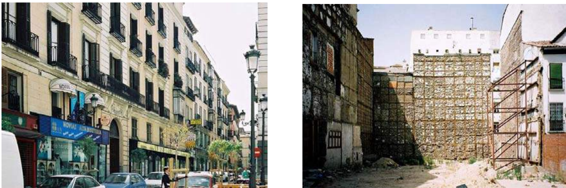
Figure 2 a&b: Timber and masonry infill-frame construction near the Plaza Major in Madrid – hidden in the facades, but revealed by demolition behind.
