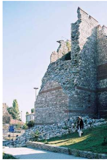
Figure 5 & 6: Istanbul City walls showing brick banding in surviving historic section and collapsed reconstructed section with fake banding.
