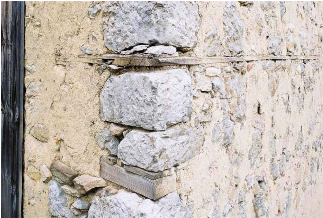
Figure 10: Laced bearing wall in Safranbolu, Turkey
