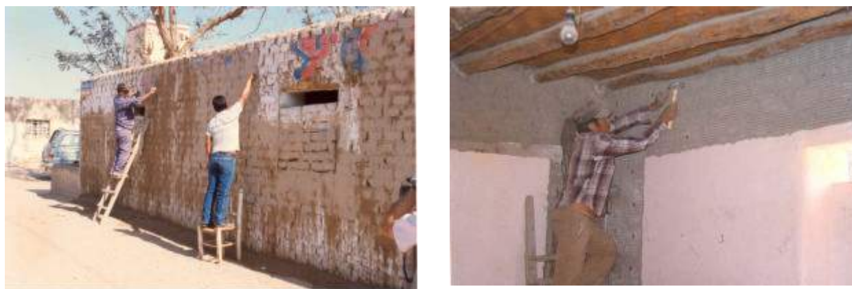
Figure 4. Adobe house in Guadalupe retrofitted in 1998 (left to right): marking horizontal strip at outside wall, nailing horizontal strip in inner side of wall.
