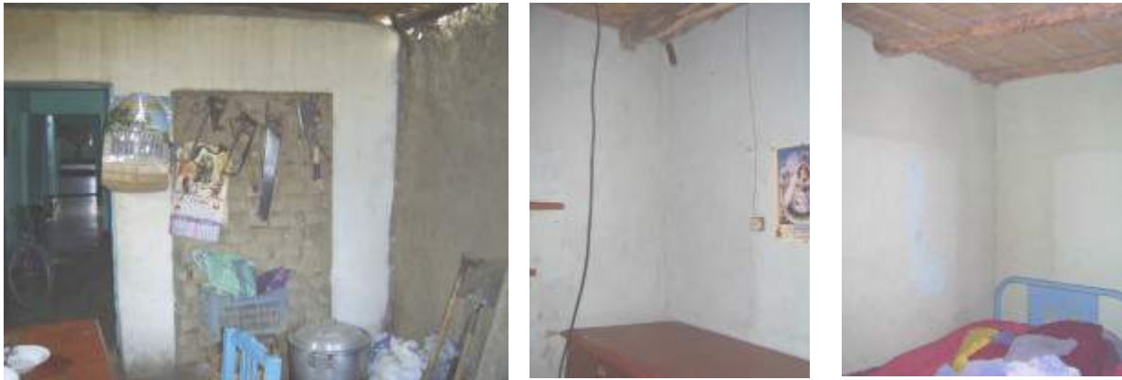
Figure 10. Pachacutec retrofitted adobe house without damage
