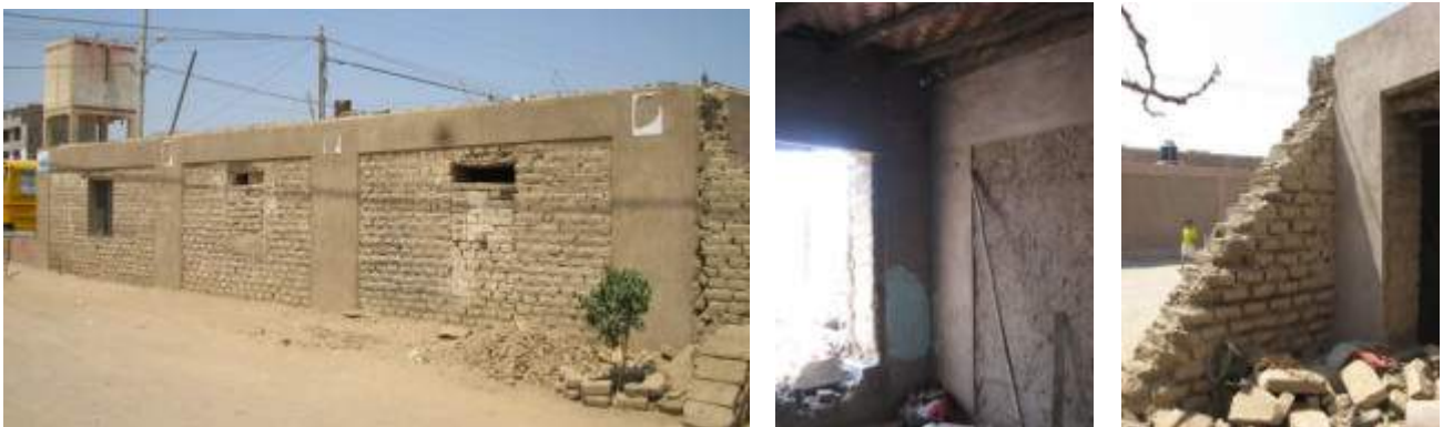
Figure 8. Guadalupe retrofitted adobe house without damage (except unreinforced patio wall)
