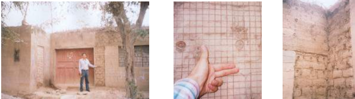
Figure 12. Partly retrofitted Parcona house without damage
