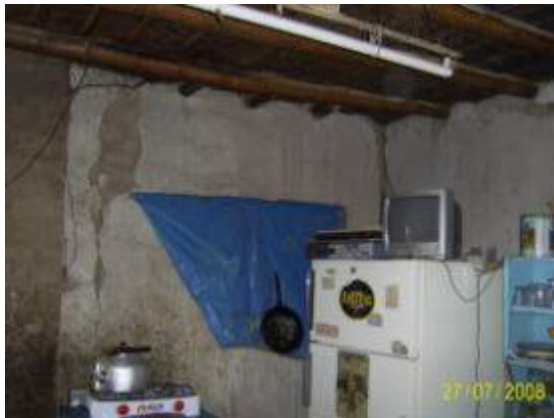
Figure 15. Non reinforced back room of the house in La Tinguiña had cracks.
