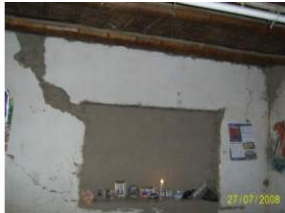
Figure 15. Non reinforced back room of the house in La Tinguiña had cracks.
