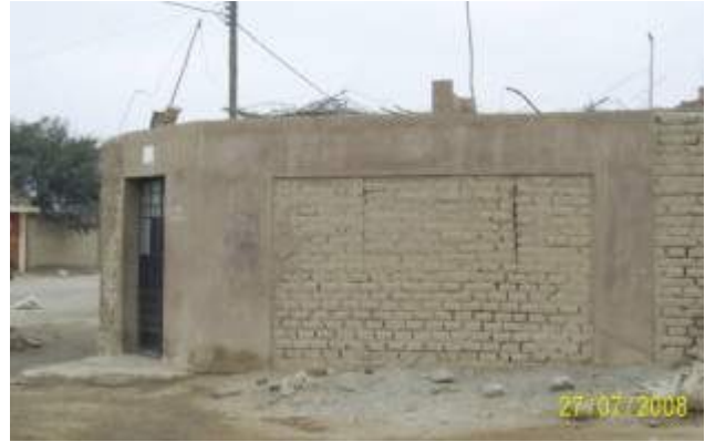
Figure 14. Partly retrofitted house in La Tinguiña had no damage.
