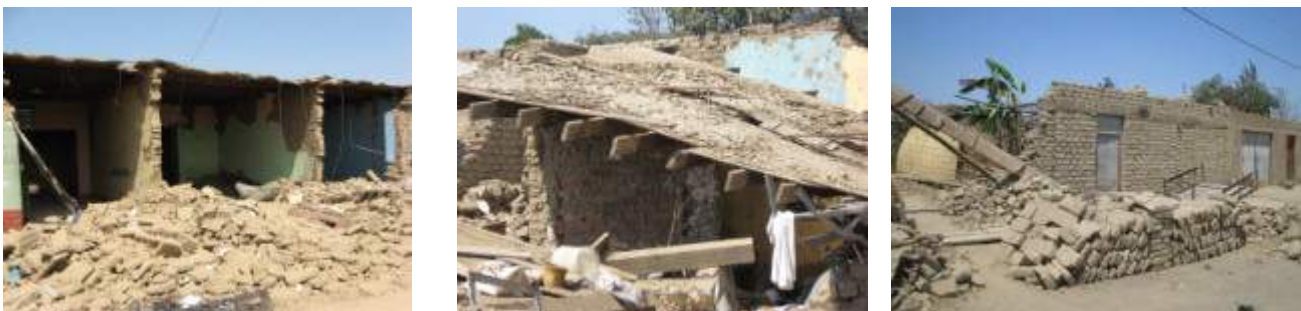
Figure 9. Other adobe houses with severe damage in Guadalupe
