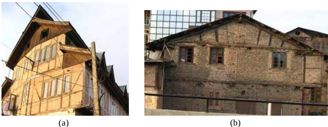
Figure 1 Traditional masonry for proven earthquake resistance: (a) Dhajji-dewari system of timber laced masonry for confining masonry in small panels and (b) Taq system of embedding timber thick walls
