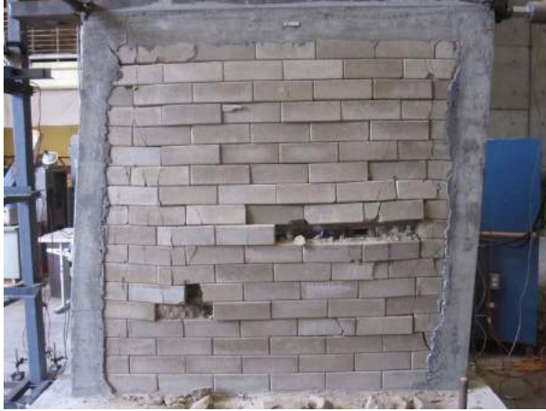
Figure 8: Wall 1, Damage at Failure
